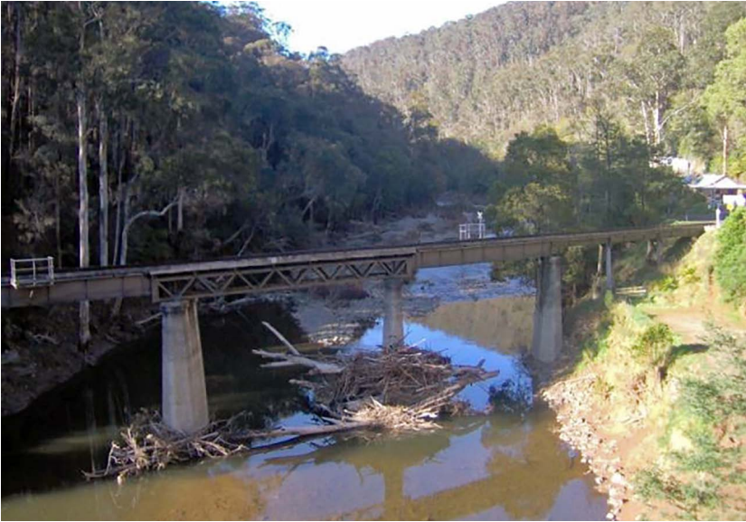
Figure 4.3: Flood debris piled up against the railway bridge to Walhalla across the Thomson River, 2008.
