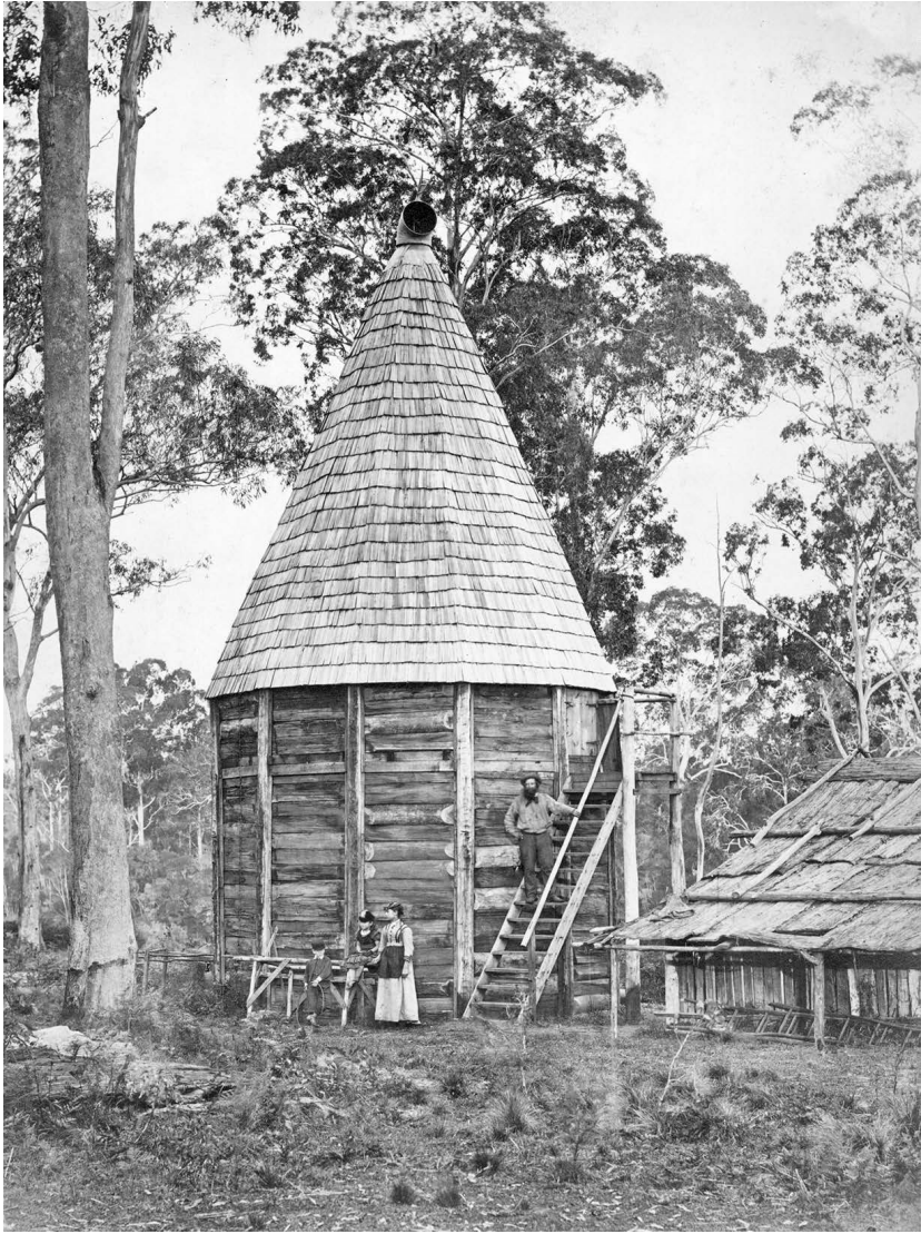
Figure 7.1: AW Howitt's hop kiln, Frederick Cornell, 1872. Hops were dried with the use of specially constructed hop kilns.
