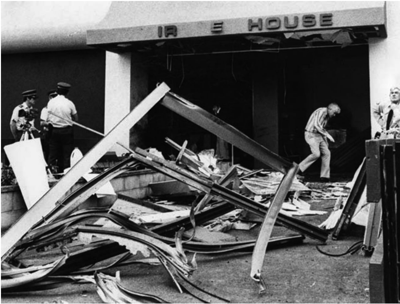
Figure 10.1: The broken front of the Wanganui Computer Centre in 1982 after the bombing.
