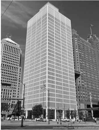
Abbildung 74. Minoru Yamasaki, Michigan Consolidated Gas Building, heute One Woodward Avenue, Detroit, Michigan, 1960–1963.
