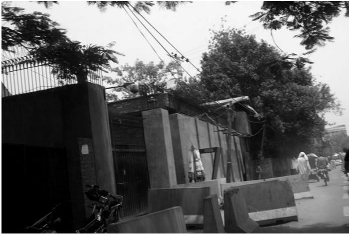
Concrete barriers and new concrete wall outside the FIA headquarters on Temple Road. Photograph by Sadia Shirazi.
