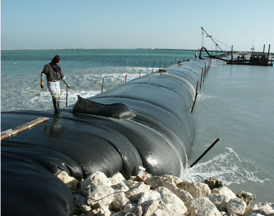
Geo-tubes being filled with sediments at a shoreline.
