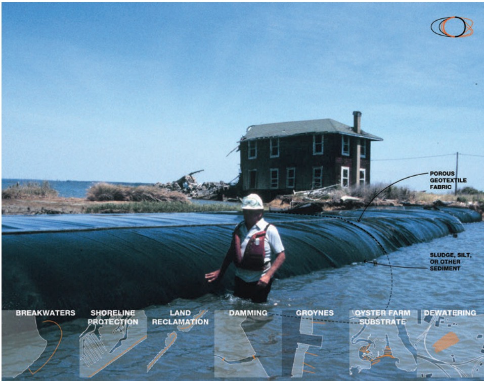
Diagram of the expanding variety of geo-tube applications. Each use implies a particular architectural character for the installation and varying relationships between water, land, and geo-tube.
