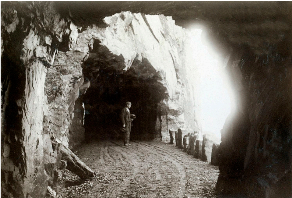
Road construction Saude-Storhjellet. Image from Road Director Hans H. Krag's photo album, 1900. Image courtesy of the Norwegian Road Museum.
