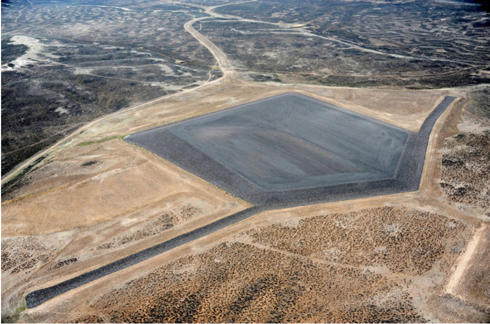
Gunnison Disposal Cell, CO.
