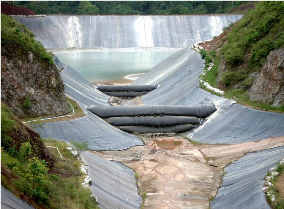
Geo-tube Dam's In Honduras. TenCate's Geotubes® have been deployed for "the construction of two dams in a river bed near a storage lagoon for mine tailings slurry in Honduras. The technology ensures storage, dewatering and filtering of polluted ground." 9
