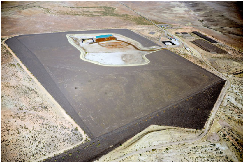
Grand Junction Disposal Cell, CO.
