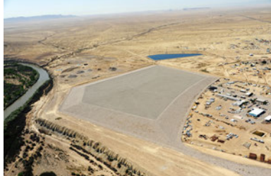
Shiprock Disposal Cell, NM.
