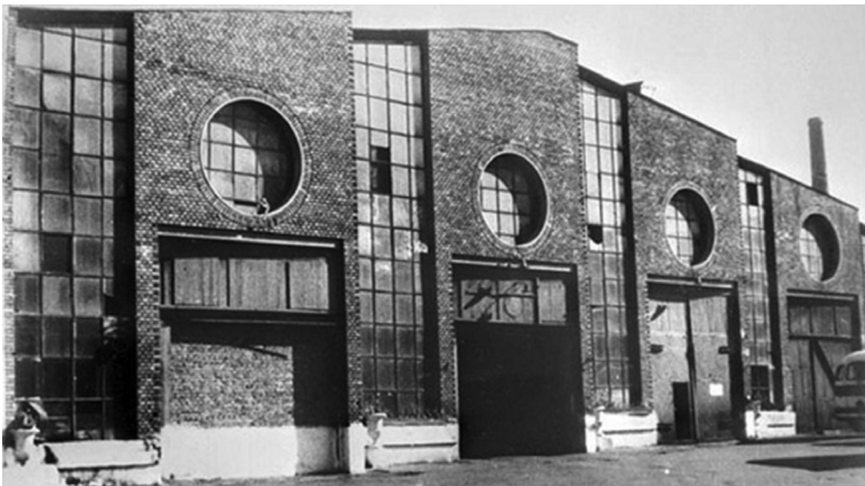
Figure 5 The Bakhmetevskii bus depot, before reconstruction.
