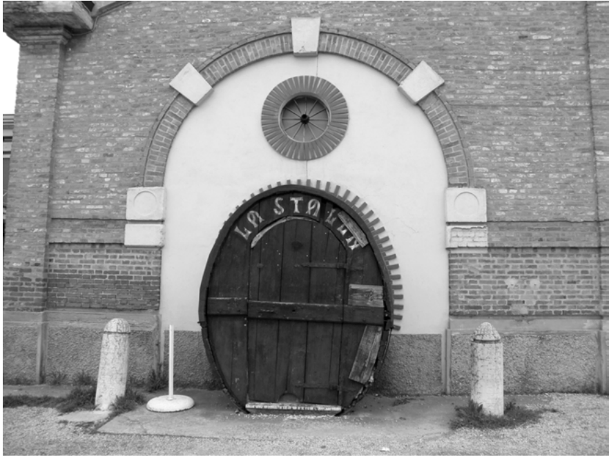
Fig. 5: The entrance to the former Pizzeria “La Stalla” in Cerese, not far from Mantua, with two cylindrical Jewish funerary pillars, reused as ornamental elements. On the right side, the one of Avraham Yedidya Basilea, brother of the Mantua kabbalist, Avi’ad Sar Shalom Basilea, who passed away in 1748, in July. On the left side, that of Avraham Ḥayyim Norsa, who died in 1783, both leading Rabbis in Mantua during the 18 th century. Despite my efforts to obtain permission to bring the funerary pillars to the Jewish community in Mantua, with the intention to putting them in a museum, together with other Mantua maševot of the 16 th –18 th centuries, the two pillars remain, up to now, at the place where the picture was taken.
