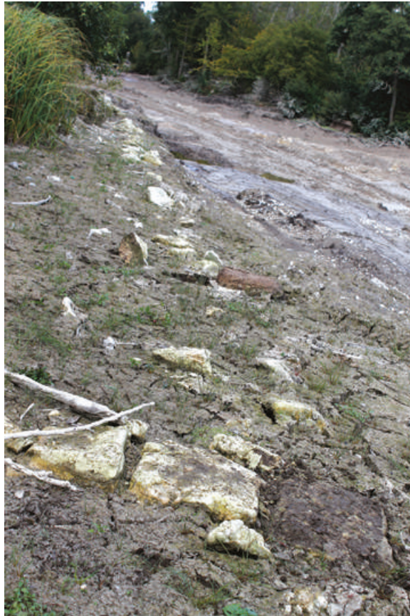
Fig. 1.2 Photograph of boundary wall of the first Fonthill House, revealed during dredging of Fonthill Lake.
