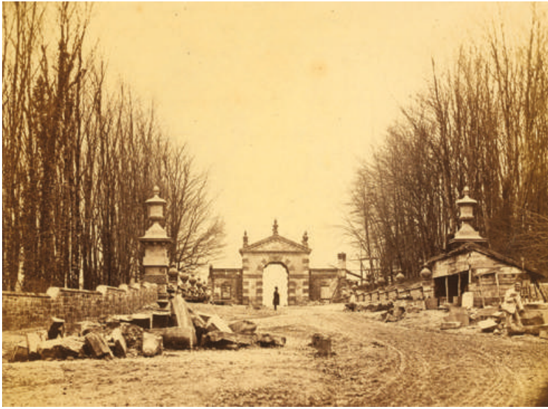
Fig. 6.29 George Devey, 'Work to retaining walls of north archway at Fonthill Bishop'.
