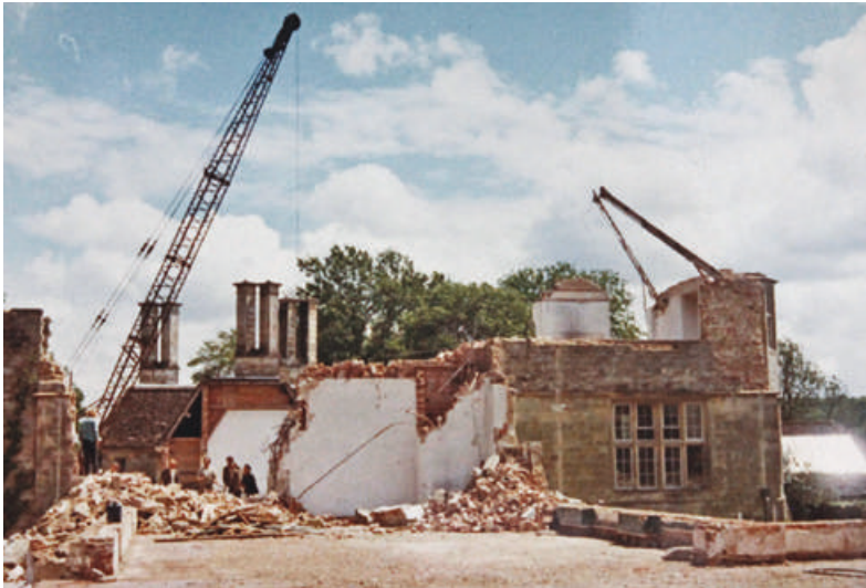
Fig. 7.11 Demolition of Fonthill House.
