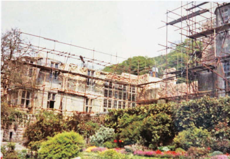
Fig. 18.10 The house during demolition in 1972. The large window in the centre lit the Hall.
