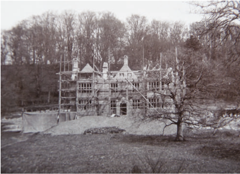
Fig. 18.4 Little Ridge under construction: the old Berwick St Leonard Manor House being rebuilt on its new site.
