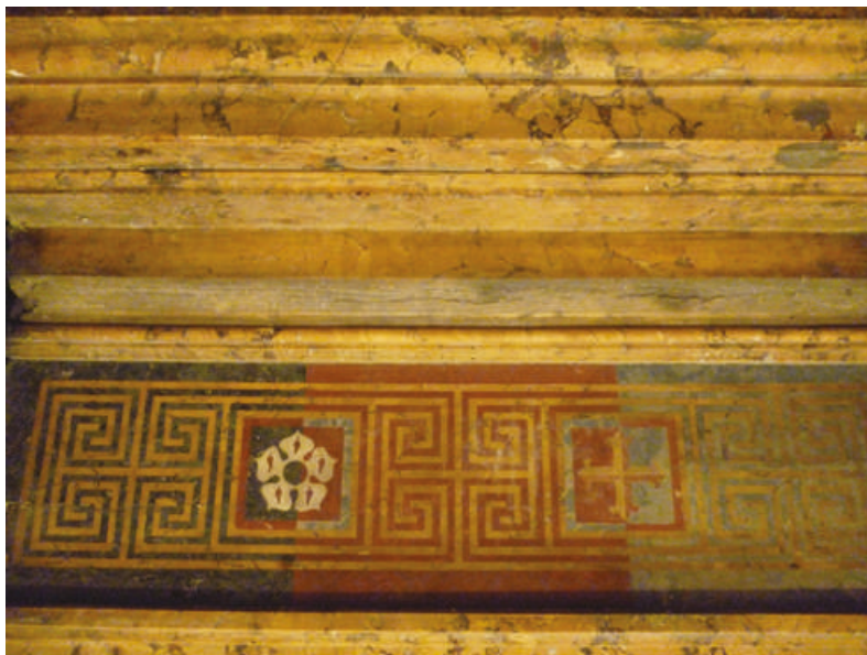
Fig. 4.14 Plaster cornice from Fonthill House, Beckford's Tower and Museum.
