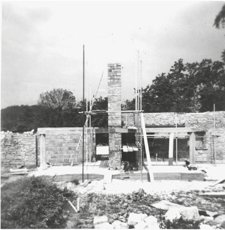
Fig. 19.3 Upper Lawn under construction looking north.
