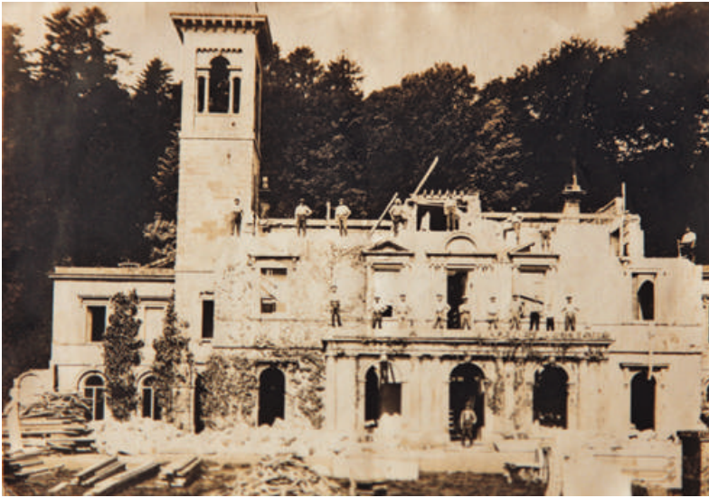
Fig. 7.6 The demolition of Fonthill House (the old Pavilion).
