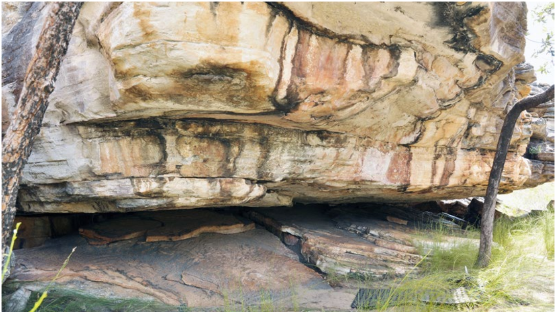
Figure 13.6 Eastern wall showing evidence of ceiling collapse at ground level, looking northwest.
