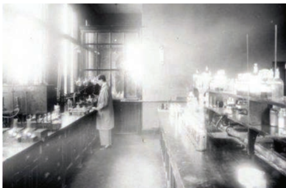
Figure 1.2 The Davy Hulme Sewage Works Laboratory, where the activated sludge process was developed in the early 20 th century (photo: United Utilities).
