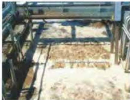
Figure 18: VRM Membrane Filters
