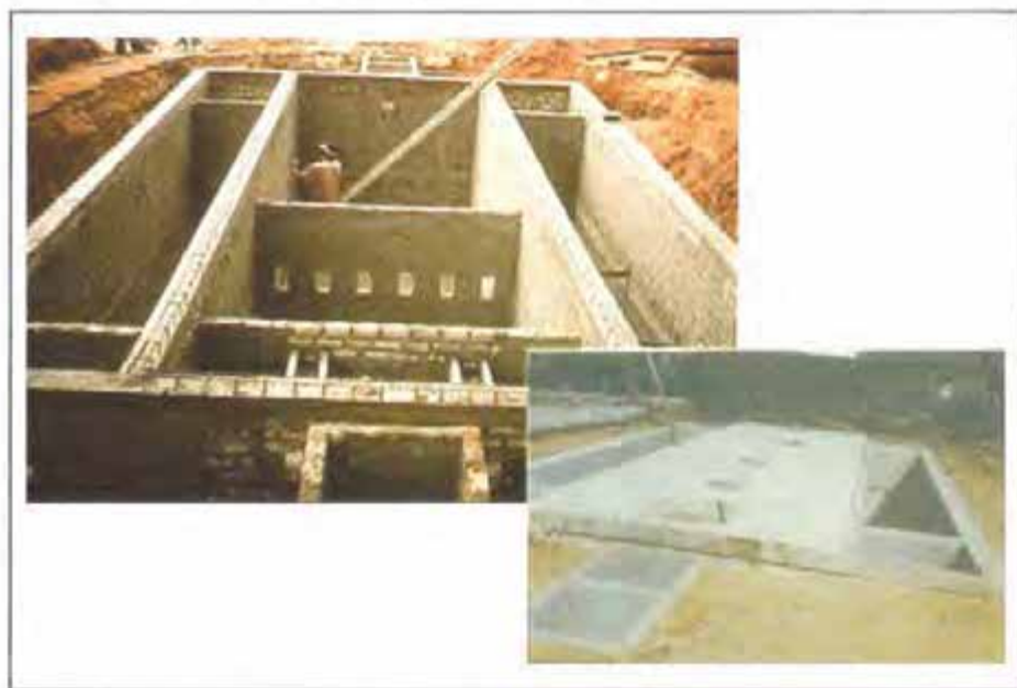
Figure 7: Photos of an Anaerobic Filter During Construction
