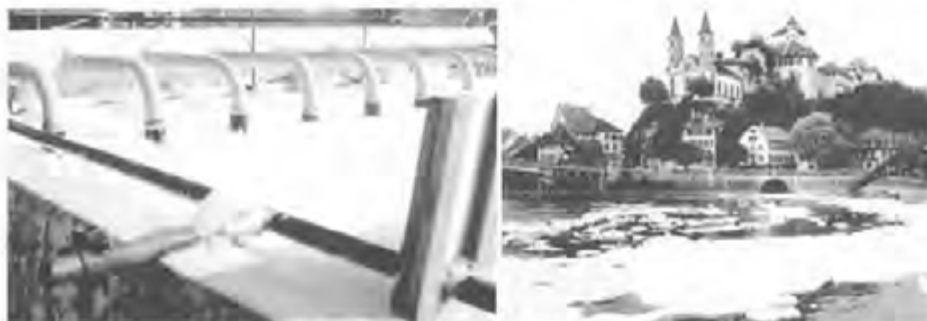
Figure 6: Excessive foaming in an aeration tank (left) and in receiving waters (right) due to nonbiodegradable detergents (branched alkylbenzene sulfonates). Pictures taken around 1964 before the introduction of LAS (archive Eawag)
