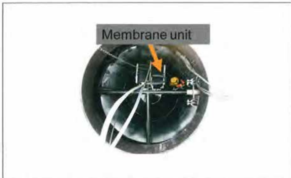
Figure 4: Upgrading of a low-tech small wwtp to a high-tech MBR system by introducing a membrane module plus aeration, Dorgeloh and Defrain (2006).
