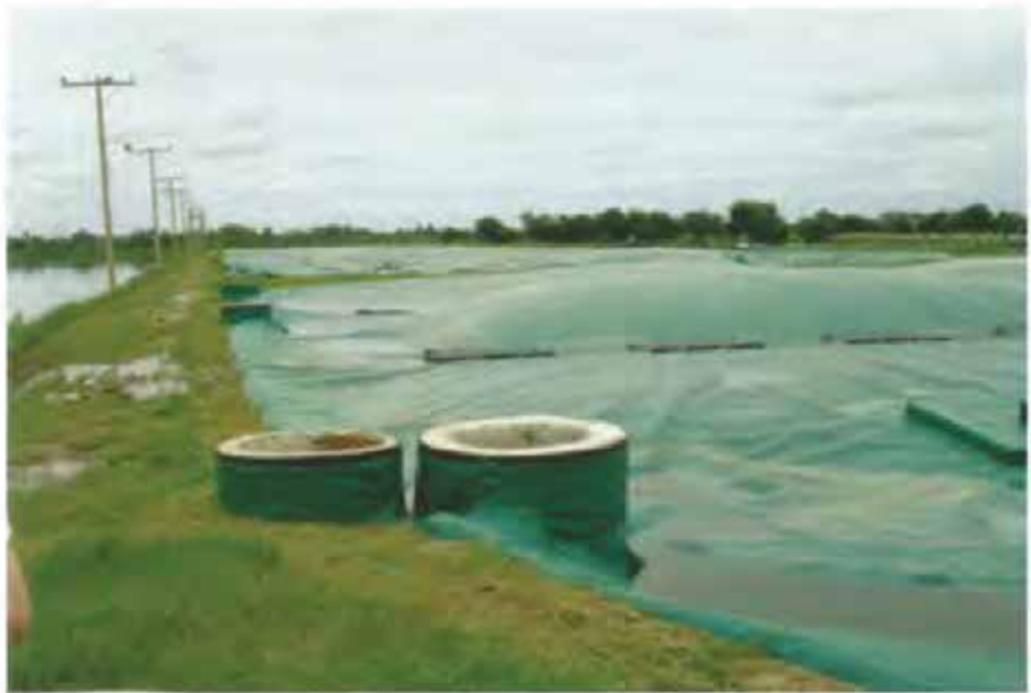
Figure 3: Covered Anaerobic Lagoons in the Industrial Wastewater Treatment Plant of Santa Cruz, Bolivia
