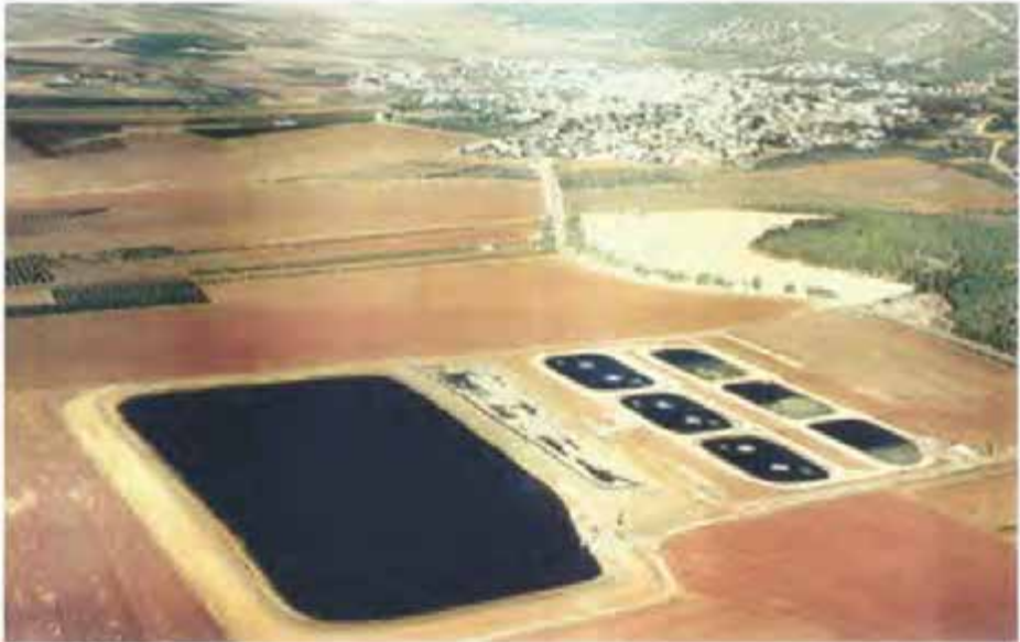
Figure 16: The Wastewater Treatment System and Stabilization Reservoir of the City of Nazareth
