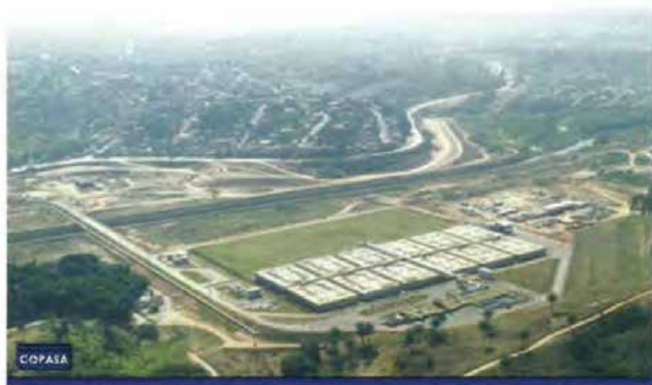
Figure 5: The Onca UASB Treatment Plant, Belo Horizonte, Brazil, Designed to Serve a Population of 1 million
