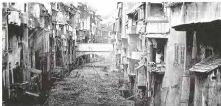
Figure 4: Drainage of wastewater along the river Birsig in Basel, Switzerland (Photo taken in 1880)
