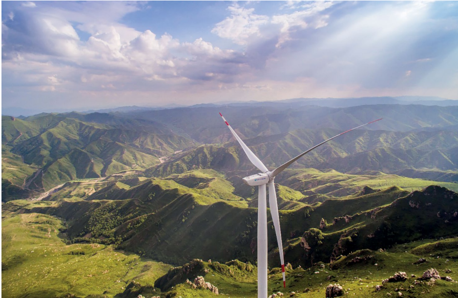
Plate 14.1 Fenghuangshan wind power plant
