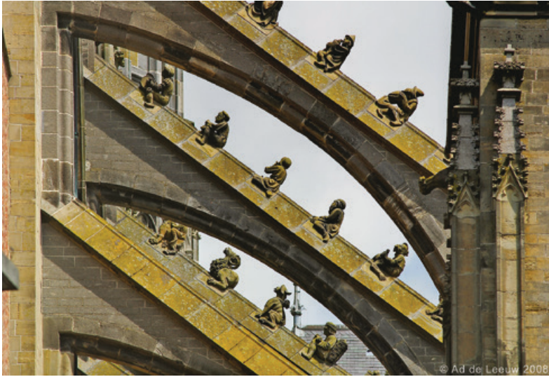
Fig. 12.4 Detail of flying buttresses of St John, 's-Hertogenbosch. Photos taken in June, 2016. Photo © Steve Whitmarsh
