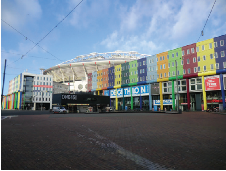
Fig 2.4 The ArenA surrounded by houses, shops and offices, Amsterdam, 2016
