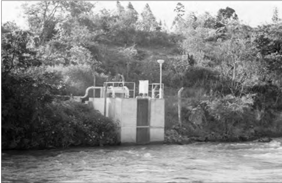
Figure 3.44: Intake structure and low lift pumping 714 .
