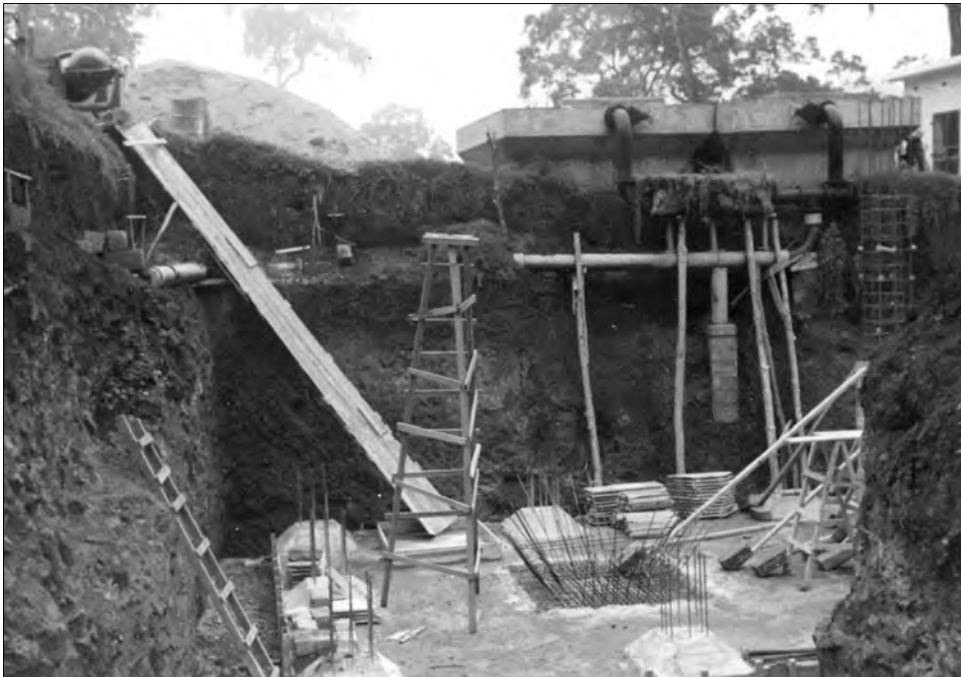
Figure 3.56: The construction of treatment works
