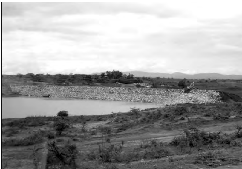
Figure 3.27: Maruba Dam site in 1983 602 .
