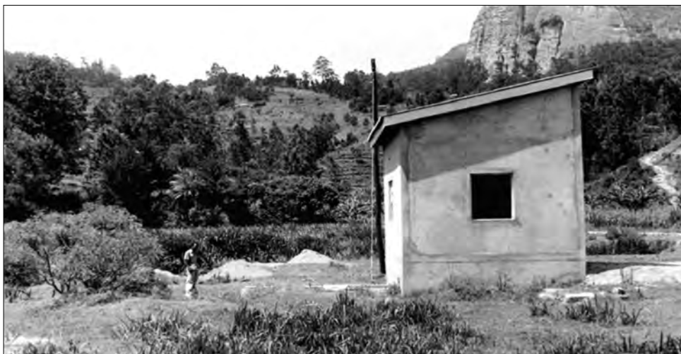
Figure 3.15: Wundanyi water project 1983 288
