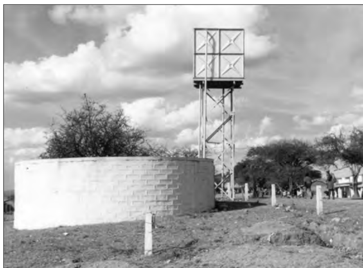
Figure 3.35: Storage tank from where water was distributed by gravity 687
