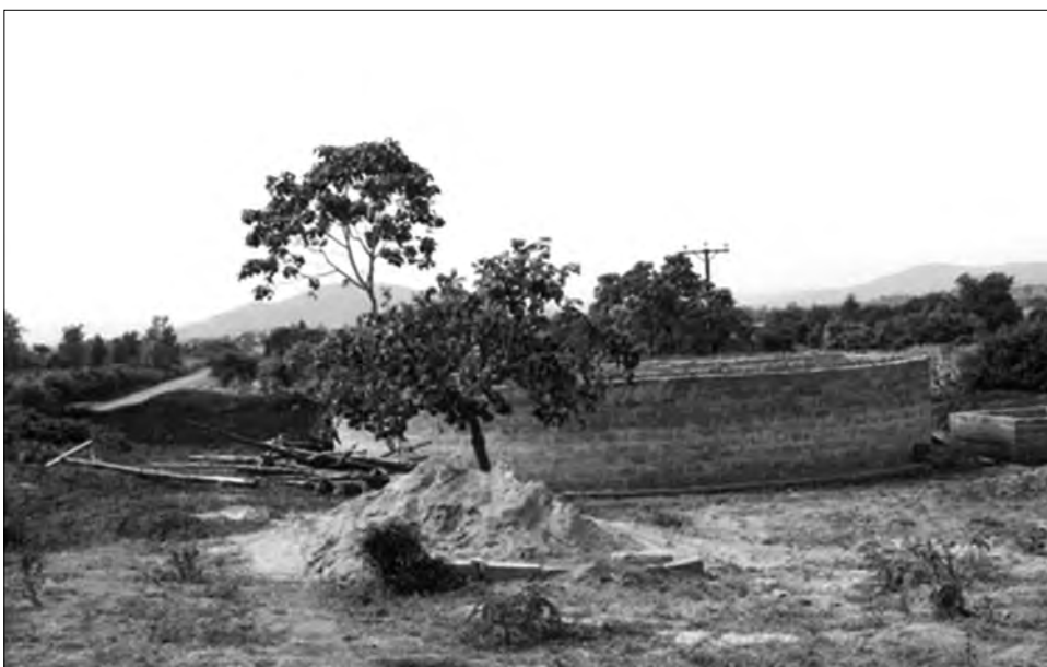
Figure 3.34: An underground block storage water tank with a capacity of 300m 3 in Sagana in 1983 666
