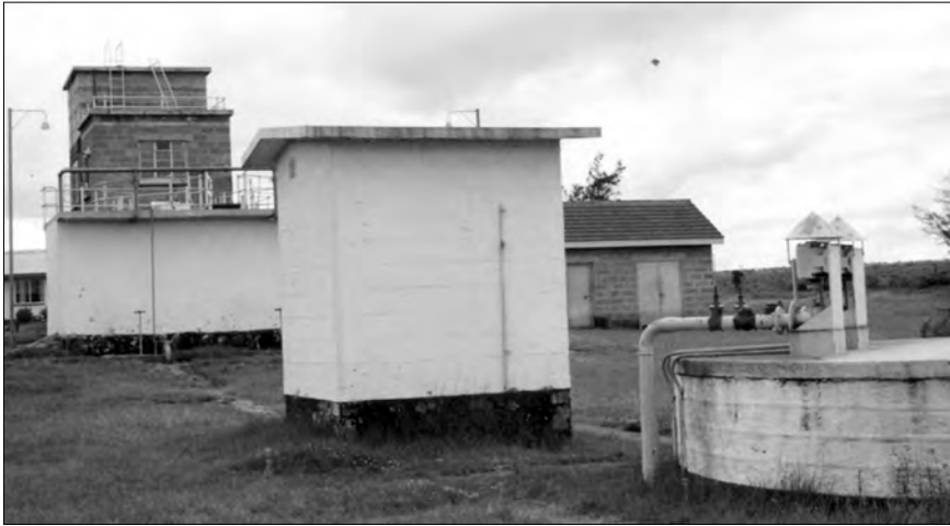
Figure 3.21: Naivasha full treatment at the existing scheme by 1983 332
