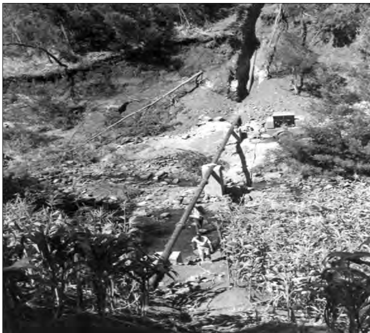
Figure 3.4: A pipe bridge constructed to withstand floods 61
