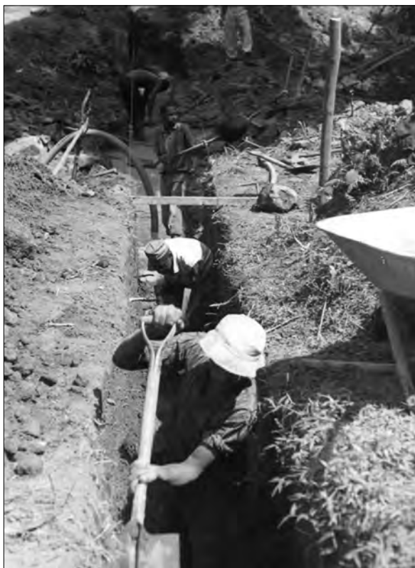
Figure 3.47: Communal labour being used to provide water supply 764 .
