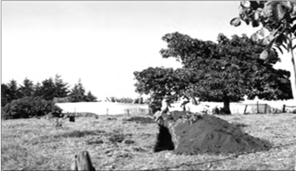
Figure 3.31: Trenching for the 8-inch pipeline leading to the main reservoirs in 1983 660 .
