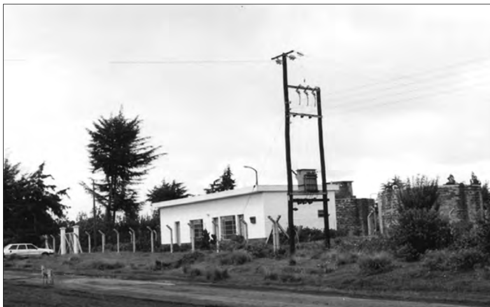
Figure 3.40: Utility building, two storage tanks, aerator and electricity supply for Limuru water supply in 1983 699 .
