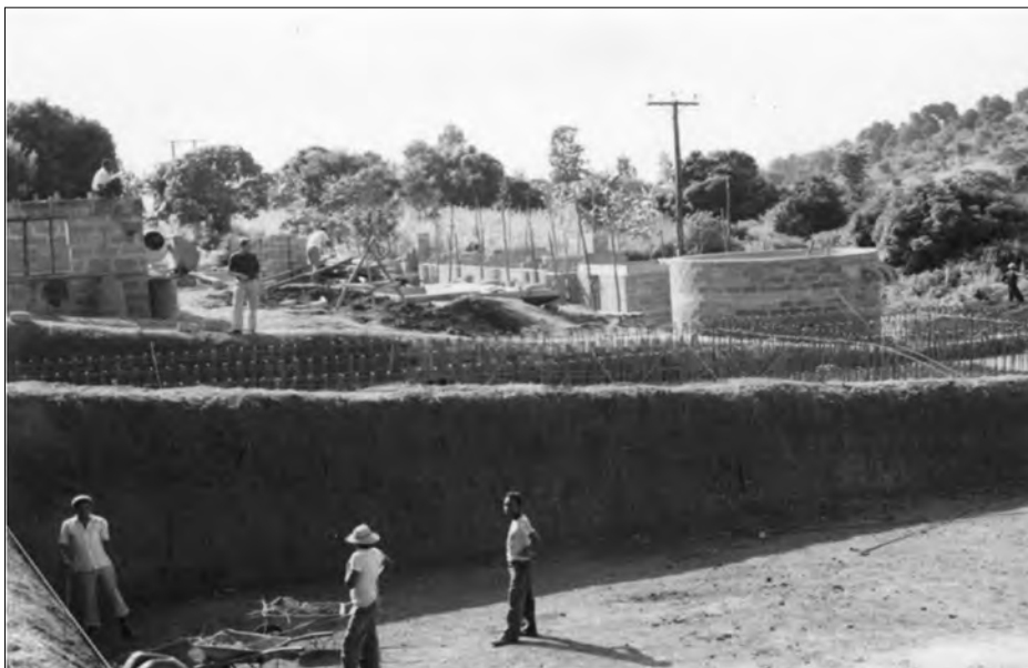
Figure 3.32: Sagana treatment plan under construction, slow and sand filter excavated in 1983 664
