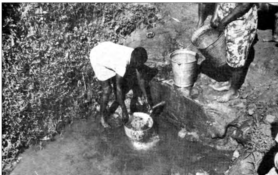
Figure 3.3: A protected spring widely used as the first stage in the improvement of rural water supplies. The concrete work prevented surface pollution of the source. However, users still covered long distances to collect water 45 .
