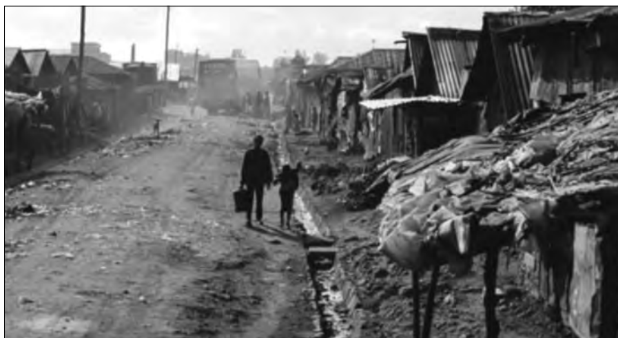
Figure 3.60: A section of Kibera slums in the year 2008
