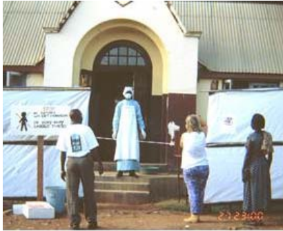
a. Main entrance of Gulu General Hospital.
