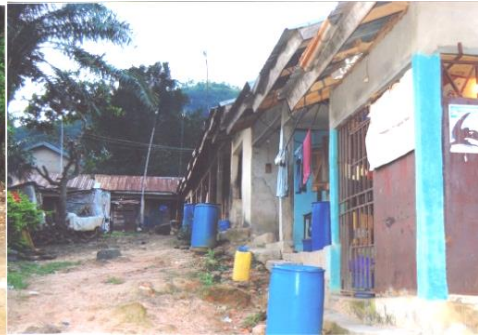
Figure 4: Typical slum house type
