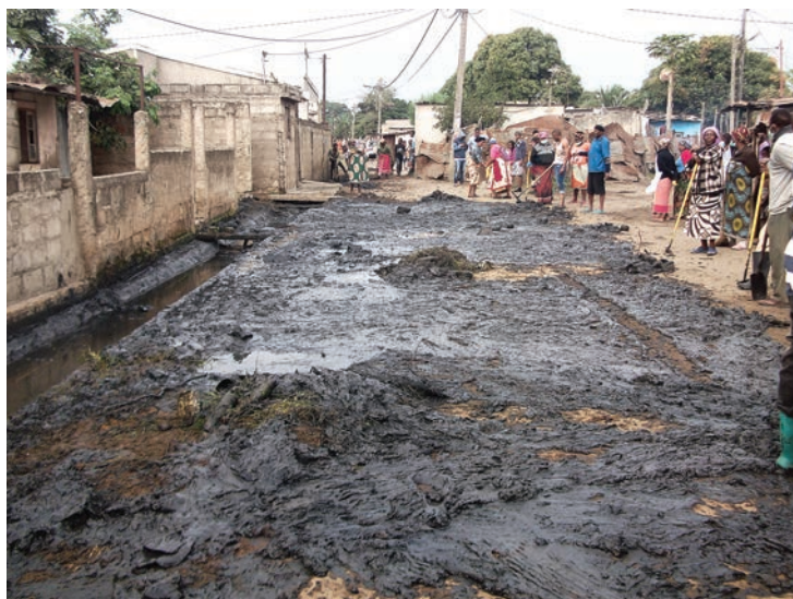
Photo 22 The sludge removed from the drainage channel.
