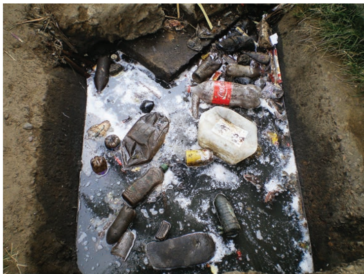
Photo 18 Waste collection is deficient. Containers overflow, so residents dump rubbish in the drainage channel.
