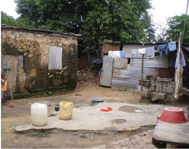
Photo 3 The original houses were built of reeds, corrugated iron or rubble and plaster. Often several households share the same yard, washing facilities and latrines.
