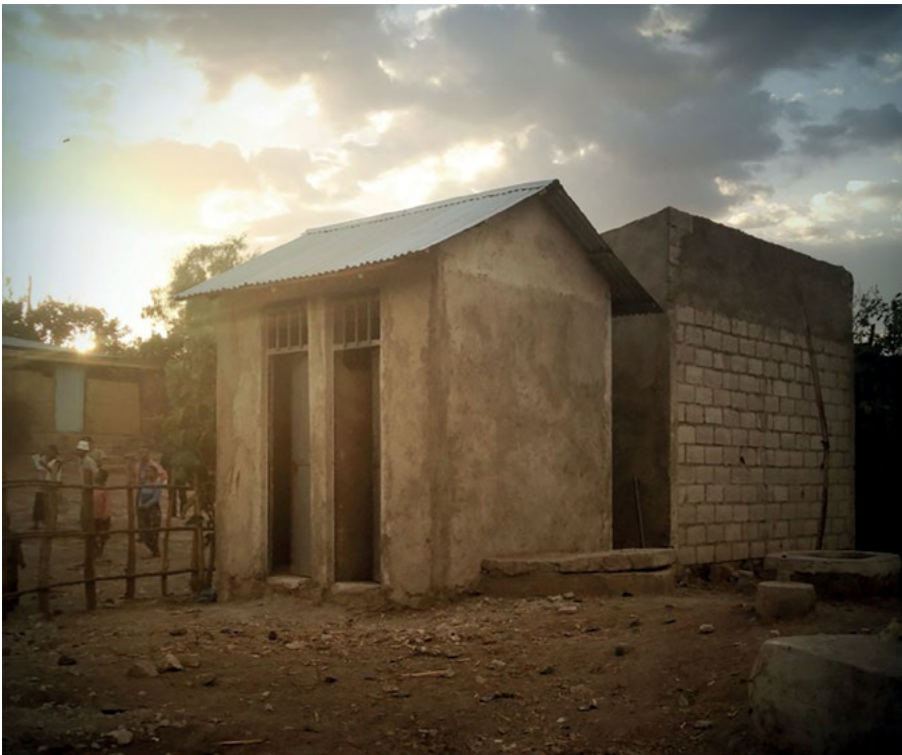
Figure 18.1 The biogas compound. The foreground building contains the latrines and the adjacent building is the community kitchen.
