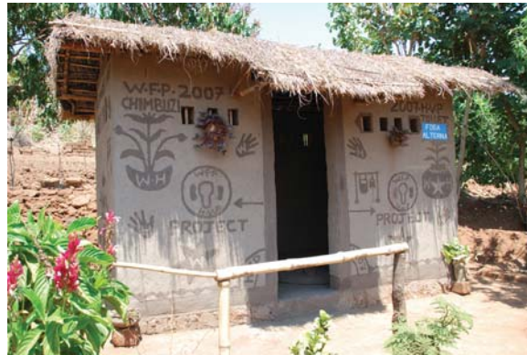
Figure 12.1 An Fossa Alterna latrine – an example of an ECOSAN latrine in Malawi.
