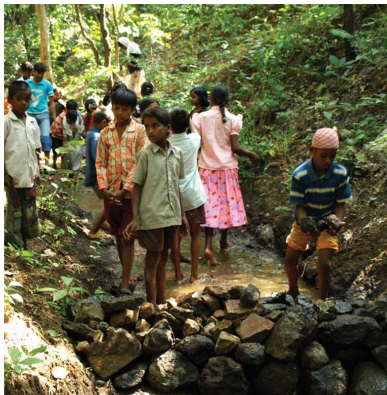
Stream erosion prevention and soil conservation work, Baripada ICCA, near Pune, India: village children learning by doing at an early age
