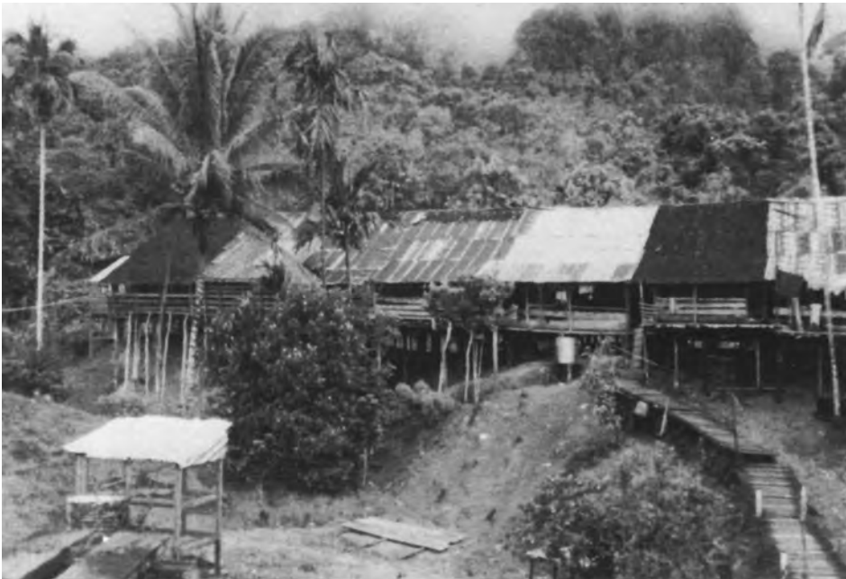
Views of a Lahanan longhouse and its communal veranda
