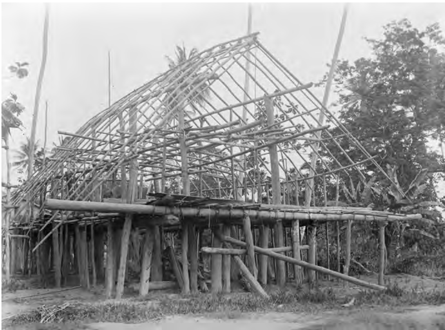
Figure 51. Framework of a new longhouse at Iasa (VKK 248: 77)
