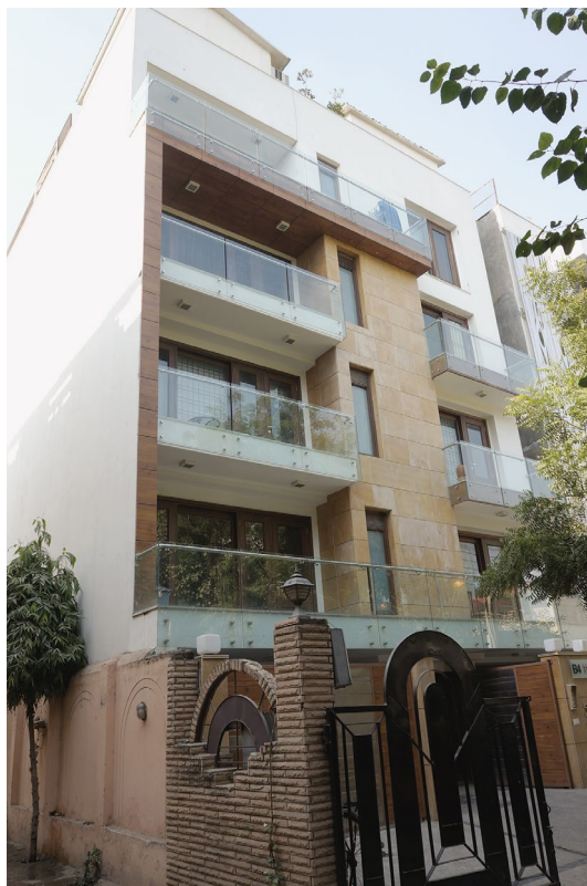
Figure 1: Newly constructed building in Safdarjung Enclave, 2013, South Delhi.
