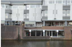
Terrace facing waterside at Middelburg, exterior and interior. Caso.
