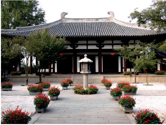
Fig. 2. Jianzhen Monk Memorial Hall in Yangzhou, designed by Liang Sicheng in 1963, and built in 1973.
