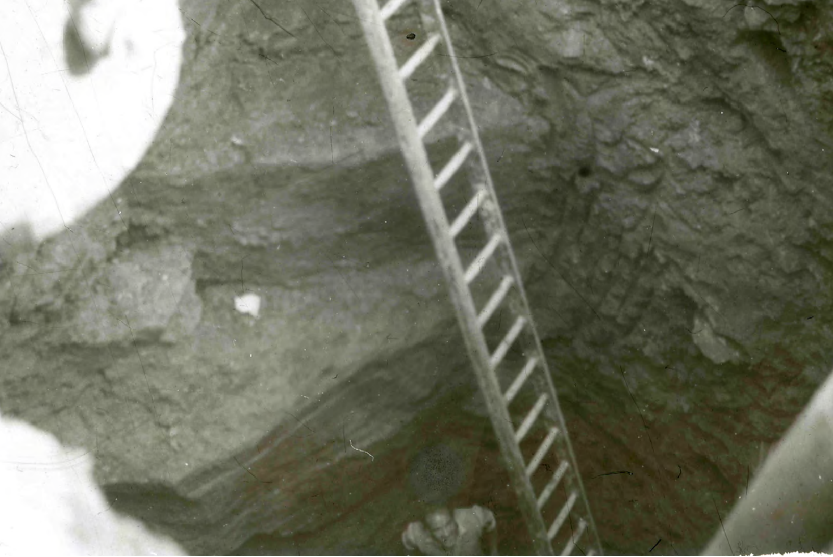
Figure 5.4: Foundation shaft H23 photographed from the south-west with a view of the moat cut. A workman is visible at the bottom giving an indication of working conditions on site that were faced by archaeologists as well as construction workers. Courtesy of Museums Sheffield.
