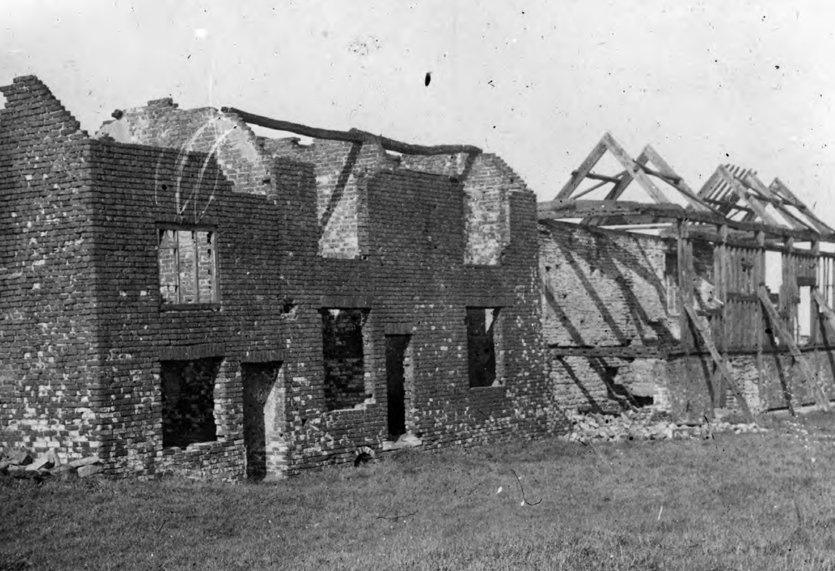
Figure 9.22: Cottages built into the ruins of the long gallery. Within a few years the brick cottages on the left were demolished and the Tudor timber framing to the right was removed. With thanks to www.picturesheffield.com (s05244).
