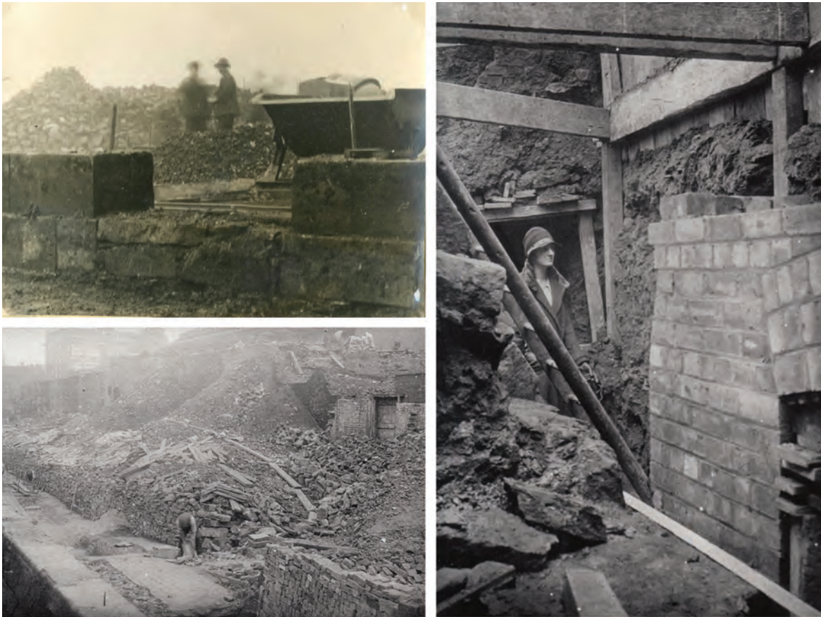
Figure 2.16: The site of Sheffield Castle during construction work 1927–30. Armstrong and Himsworth experienced considerable difficulty recording archaeology on an ‘active’ construction site. The right-hand photograph shows the wattlework believed to be Anglo-Saxon (next to the woman’s hand), which is discussed in Chapter 3. This photograph appeared in Himsworth’s diary along with the top left-hand photograph showing construction work near the courtyard buildings, with a planning frame placed on the walls of one of these buildings for a foundation shaft to be dug there (see also Figure 3.17). The bottom left photograph records building work in 1930 at the north of the site above the Don before Castlegate was built. Courtesy of Museums Sheffield.
