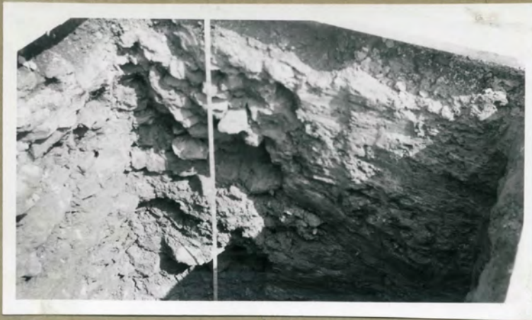
9. 93 East + North Drawbridge pier (SE end abutting on solid rock. Rubble fill L. Solid R
