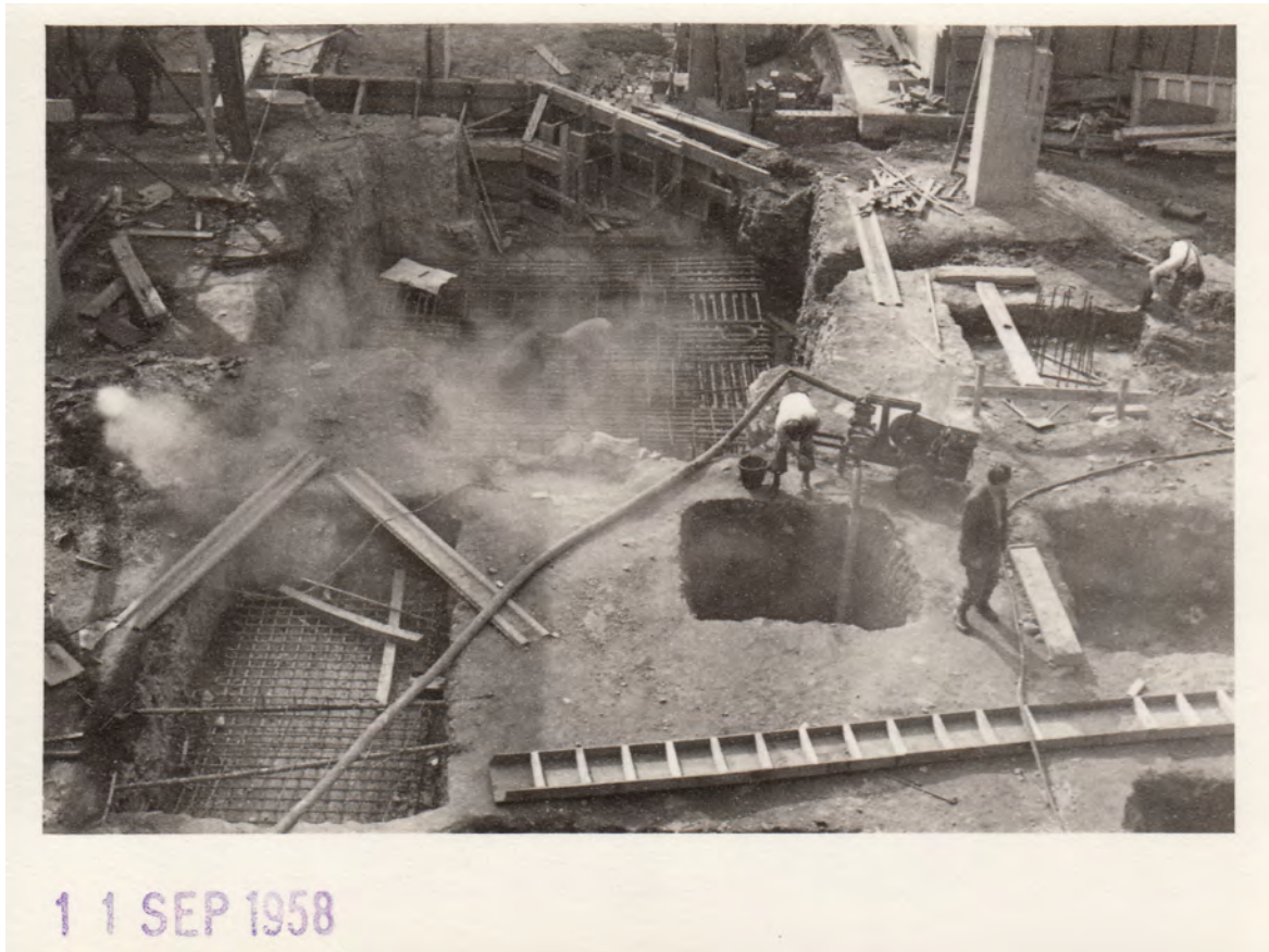
Figure 4.12: Foundation shafts being dug by construction workers. This is the 'excavation grid' that Butcher recorded. Courtesy of Museums Sheffield.
