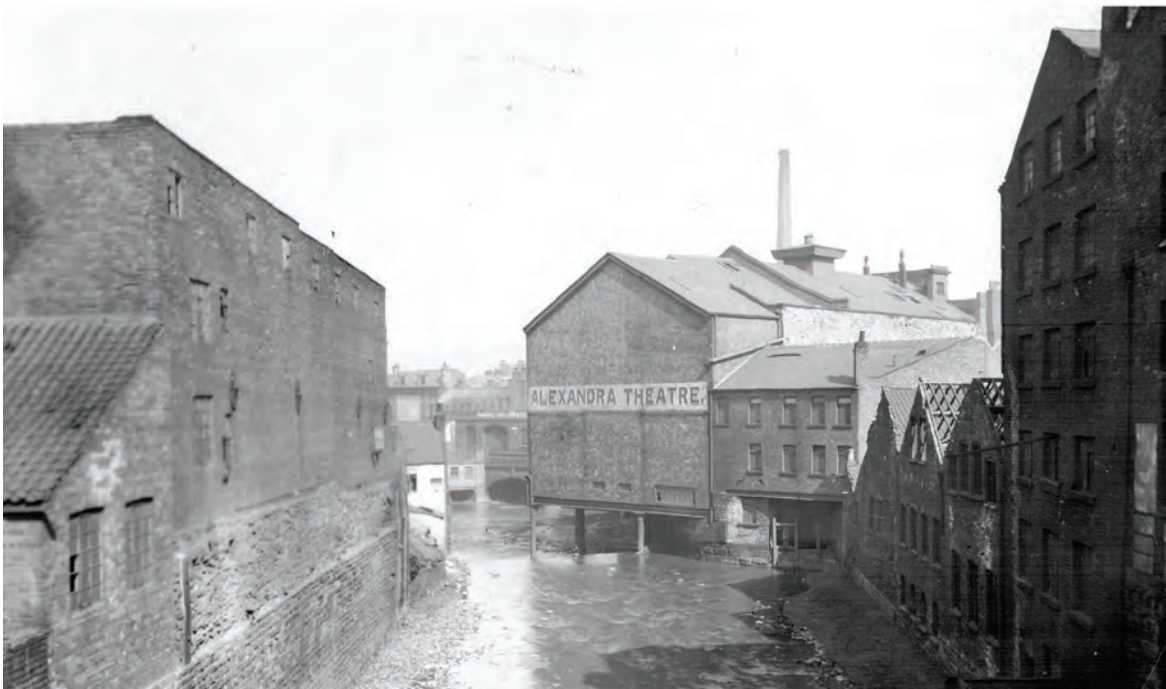
Figure 5.25: Early 20th-century photographs of the east side of Castle Hill. A photograph (top) from 1918 labelled ‘West wall of passage, but East of Castle site ... composed of stone, part dressed, part rubble, set in lime mortar’. It is noted that the wall was used ‘as a foundation for a building, now used as a slaughter house’. Another photograph in the archive, which is a close-up of the right-hand end of this wall, is labelled ‘Part of Sheffield Castle wall, discovered while pulling down old house, built in 1666, on the site of Sheffield Castle moat’, and it is said to be located opposite the weir on the Sheaf. Courtesy of Museums Sheffield. An early 20th-century photograph (bottom) showing the Alexandra Theatre and, on the opposite bank of the Sheaf, a white building which may be what Butcher described in his 1972 typescript as an “irregularly shaped house” ... which is brick-built and seemingly of 18th-century date but has what appears to be a masonry wall at its north-east corner’. With thanks to www.picturesheffield.com (s12223).
