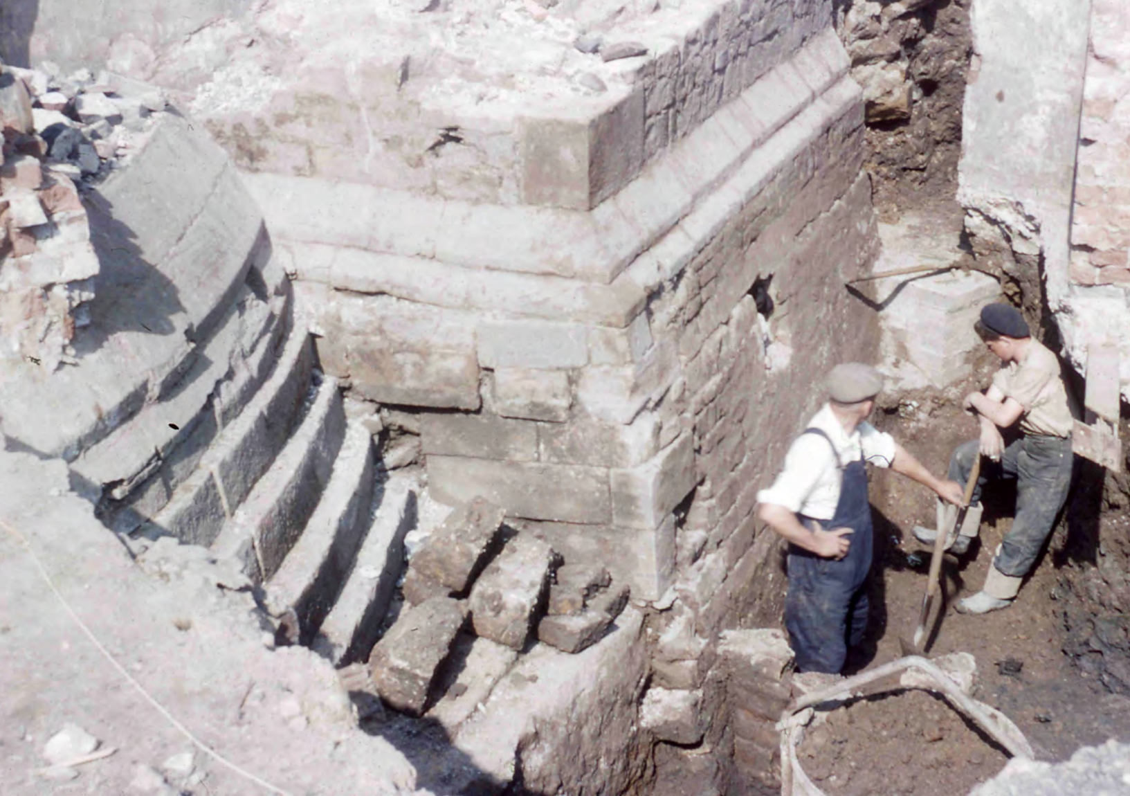
Figure iv: Construction workers digging a foundation trench next to the remains of the gatehouse of Sheffield Castle in the late 1950s. Courtesy of Museums Sheffield.
