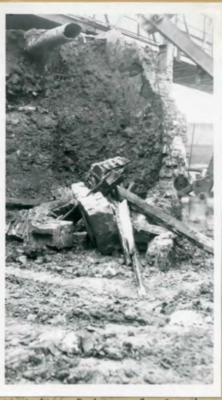
47 Filling behind B & C ret. wall appears to have carried away upper part of slope of moat seen in T.H.C (see 17)
