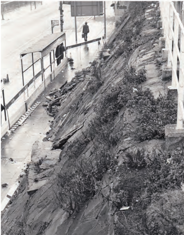
Figure 1.16: Collapse of the retaining wall above Castlegate in 1972. A section of castle wall is visible above the right-hand end of the bus stop (top) and another at the lower part of the slope (below). Recording of these exposed parts of the castle was undertaken by Pauline Beswick of Sheffield City Museum. Courtesy of Museums Sheffield.
