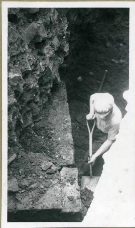
H.2-4. from N.E NE angle of drawbridge pier, destroyed to ashlar coarse rubble filling above
