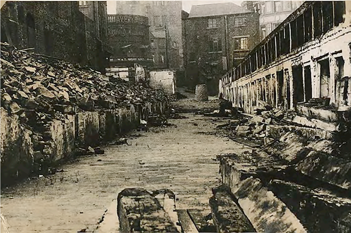
Figure 3.5: Demolition of the slaughterhouses along the bank of the Don. A photograph from the diary of Joseph Himsforth. Their removal allowed him to record the north side of the site. At the bottom right are the timbers that Himsforth believed had been reused from the castle. Courtesy of Museums Sheffield.
