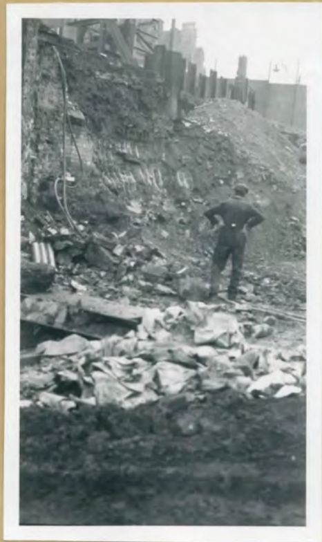
46 Corner of piling before ← Warrgate/Exchange St ditch exposed
