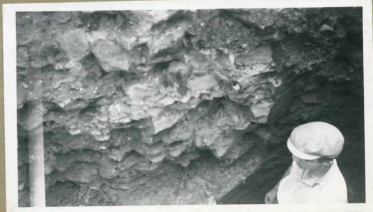
10. H2-4 from N Rubble fill (includ- ing water worn boulders) behind ashlar face (remnant beyond head of figure.)
