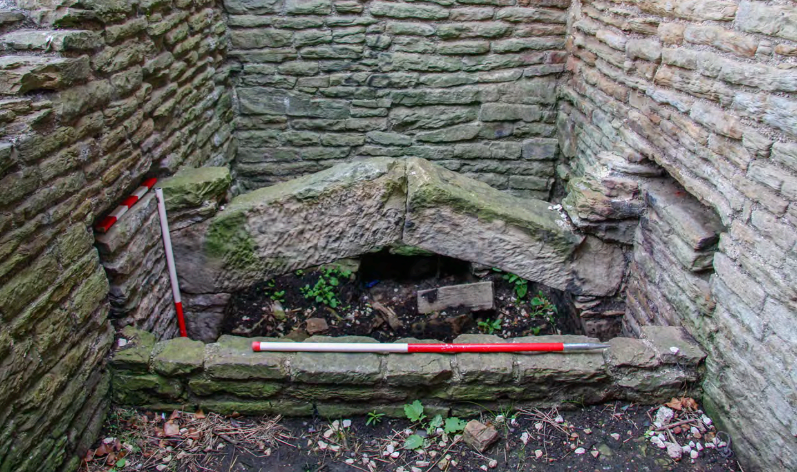
Figure 8.16: The garderobe in the three-storey tower. It takes the form of a low stone arch across the room; there was an associated timber structure and a drain leading through the north wall. Wessex Archaeology.
