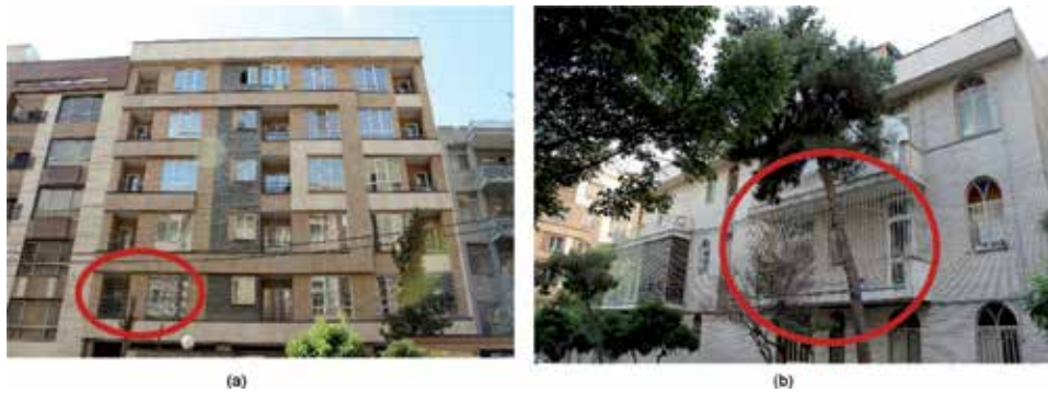
Figure 12. (a) Southern apartment. (b) Northern apartment.
