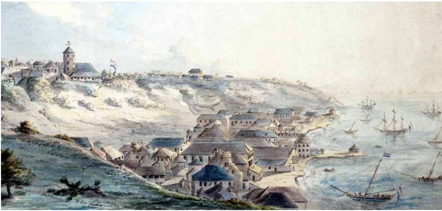
Figure 13.1: Lower Town as it appeared in 1774. Top: view to the south with the weighing house (blue roof) and the headquarters of the Dutch West India Company directly behind it in the foreground, and the Dutch Reformed Church and Fort Oranje on the cliff to the left (Source: Algemeen Rijksarchief, 4.MIKO 313).
