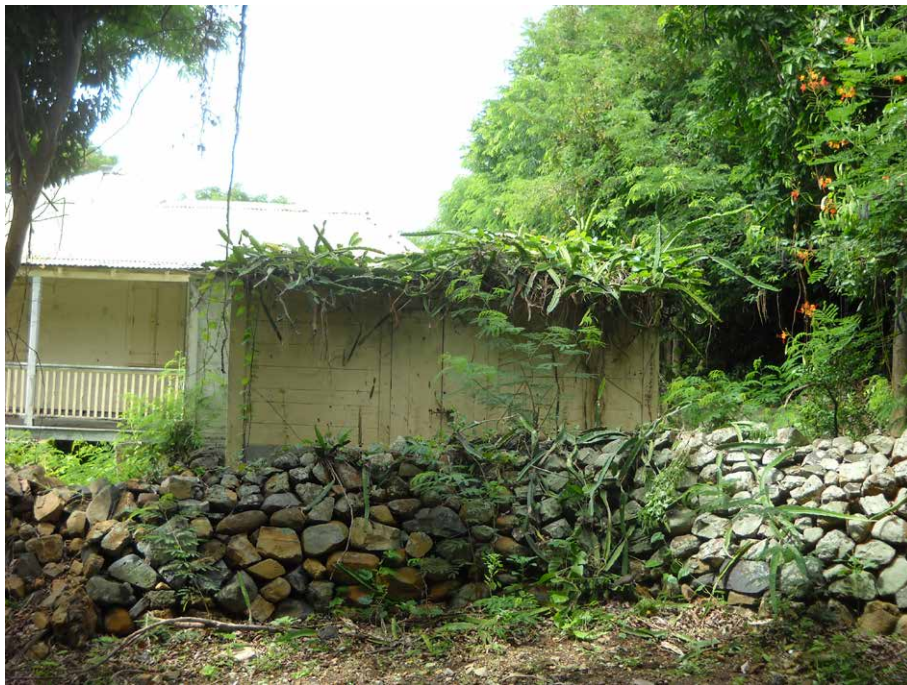
Figure 14.10: Example of the dry-stone pile boundary walls in the survey area.
