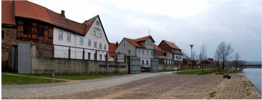
Figure 5. The city of Würth (Main River), a flood wall integrated in the historic city walls.
