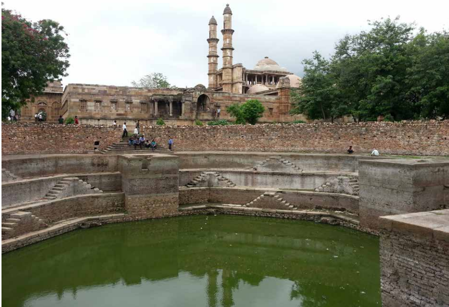
Figure 2. Another typology of a stepped water tank serving multiple uses is found at the World Heritage Site of Champaner (India).
