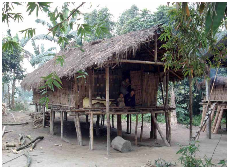
Figure 6. The vernacular housing in bamboo on the river island of Majuli (India) is built on stilts in order to protect it against regular floods.
