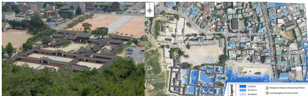
Figure 2. The temporary Palace at the Hwaseong Fortress and the flood inundation map of the site with a 100-year return period of rainfall scenario (Cultural Heritage Administration of Korea; NRICH 2009).
