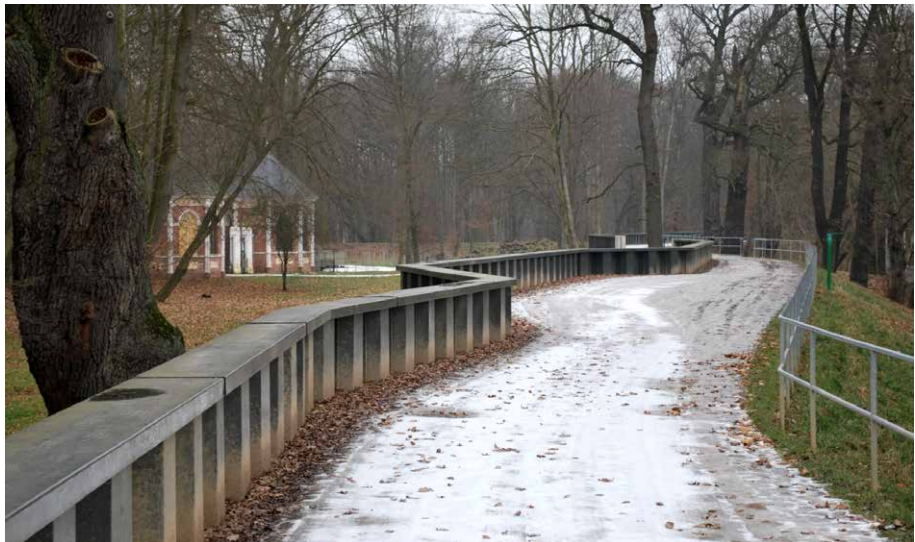
Figure 3. The city of Dessau (Elbe and Mulde Rivers), the historic garden 'Luisium' (World Heritage Site Wörlitz Gardens). a: A temporary water-filled tube solution serving to raise the protection level of the historic dike and lock its openings; b: An obtrusive stationary sheet pile wall on top of a historic dike, impairing the view of the park folly.
