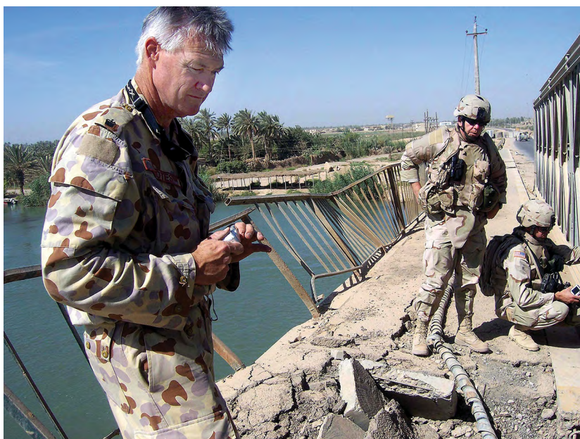
Major Cootes, Chief of Engineers on Multi-National Corps – Iraq, in 2005 surveying a bridge that was partially destroyed by a VBIED attack in 2004.
