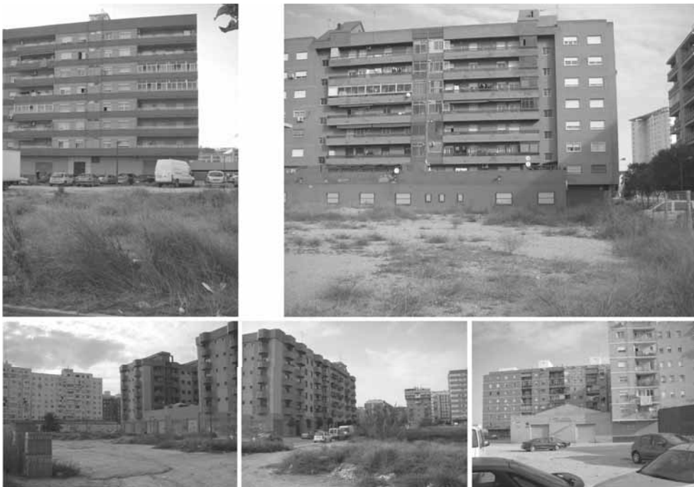
Figures 17. Examples of the periphery of the City of Valencia in the 80s: (1) Nou Benicalap; (2) Beniferri; (3-4) Orrriols; (5) Torrefiel (Copyright Demetrio Munoz, Nov 2006).
