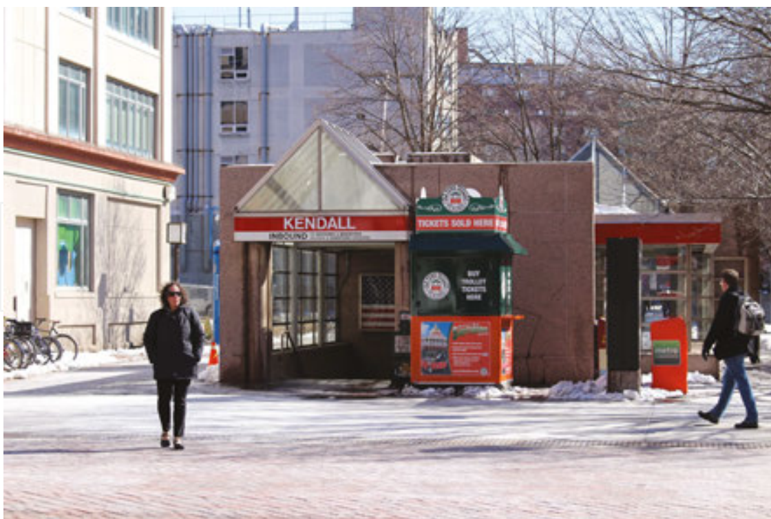
Figure 11. Transit station, bicycles, pedestrians: a walkable environment (author's picture).
