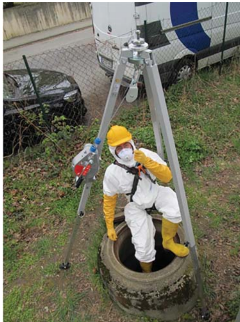
Figure 7.4 Entering the sewer network with a tripod. Source: Jakob Benisch (TU Dresden).
