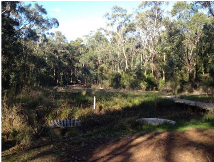
Figure 11.8 Wicks Reserve bioretention basin. Source: Jérémie Bonneau (INRAE).
