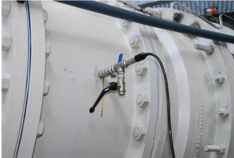
Figure 3.45 In situ constructed pressure measuring mount. Source: courtesy Kees Kooij (Deltares).
