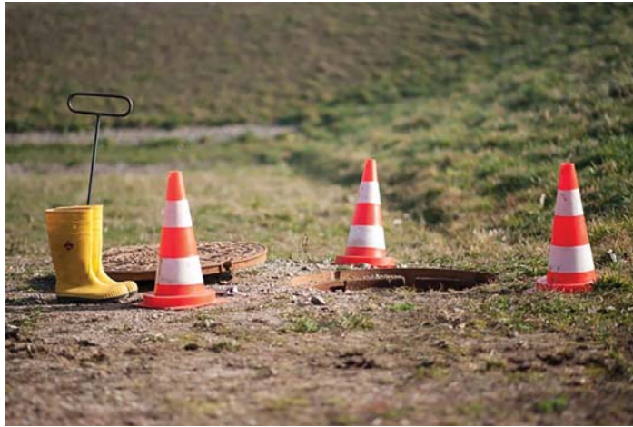
Figure 7.1 Some of the safety equipment required to enter UDSM systems. Source: courtesy of Robert Lohse Photography (2014).
