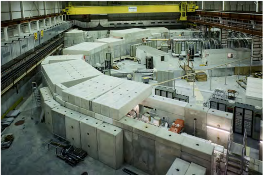
Fig. 6. The AA ring in its hall (1980–81), before and after being put under heavy concrete shield.
