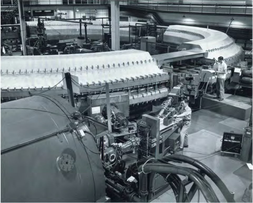
Fig. 1. The Brookhaven Cosmotron with the injector van de Graaff in the foreground (courtesy of Brookhaven National Laboratory).
