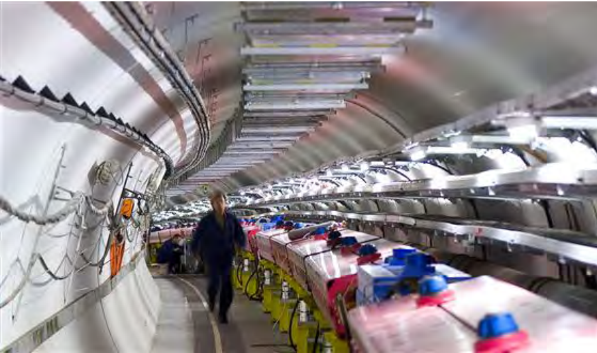
Fig. 4. Photo of the 800 m proton beam transfer line for CNGS with the tilted magnets.
