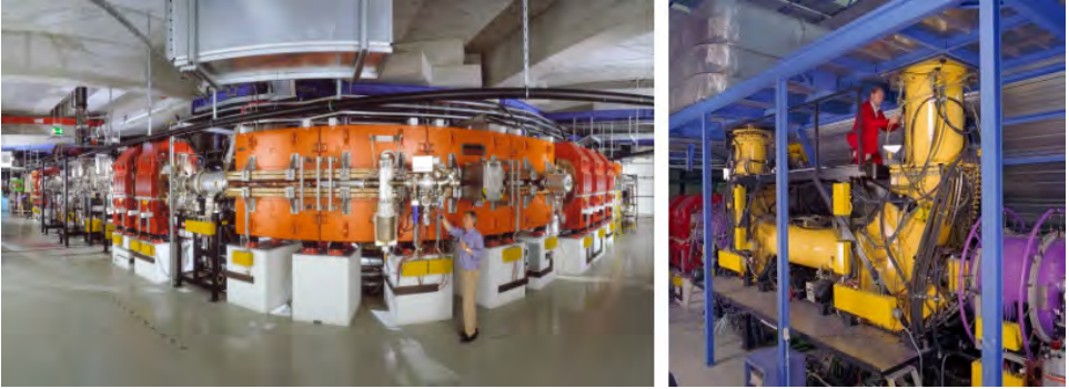
Fig. 8. Left: The picture shows the long straight section for in-ring experiments with one of the six 60° bending magnets in the foreground. Right: ESR electron cooler (yellow) between compensation solenoids (violet) counterbalancing the horizontal–vertical coupling by the cooler solenoid field.
