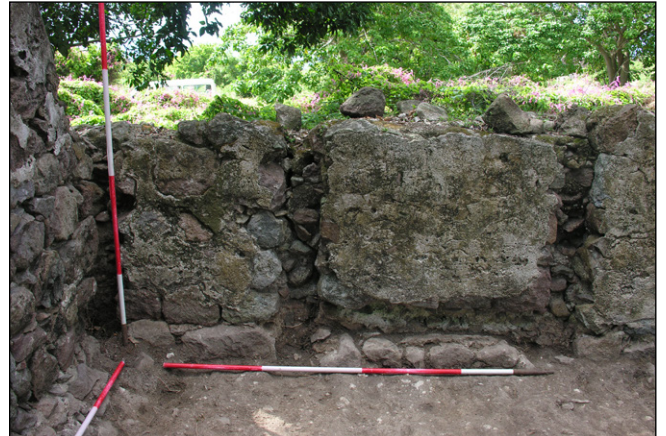
Figure 2.19. Fenton Hill: Structure A, S wall showing horizontal slot (125), linking vertical slots (126 to the left, 123 to the right), the top of the offset course to the right, and the scar of the mortar facing to the left; from N
