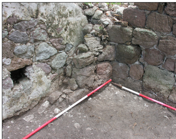
Figure 2.21. Fenton Hill: SW corner of Structure A, showing overlapping wall, and drain hole in wall, from NE
