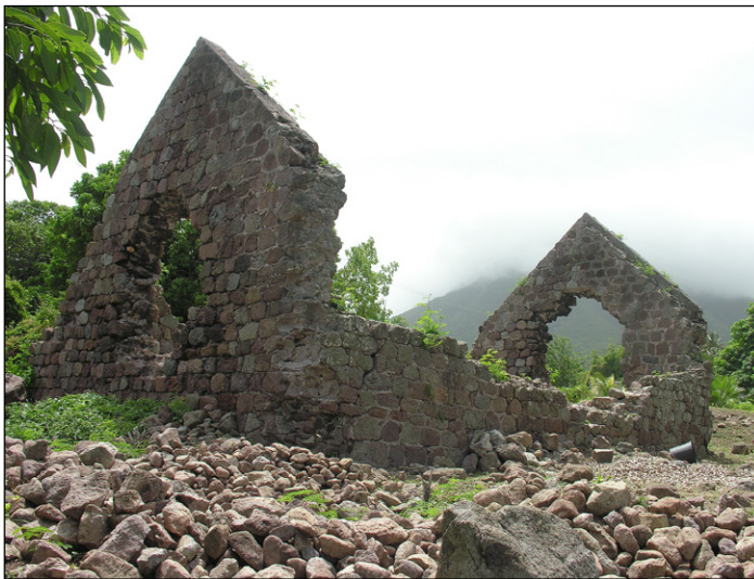
Figure 2.1. Fenton Hill: boiling house (B) from SE
