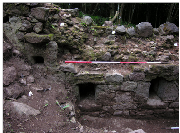
Figure 3.9. Upper Rawlins: boiling train showing stoke-hole apertures and vent above, from W
