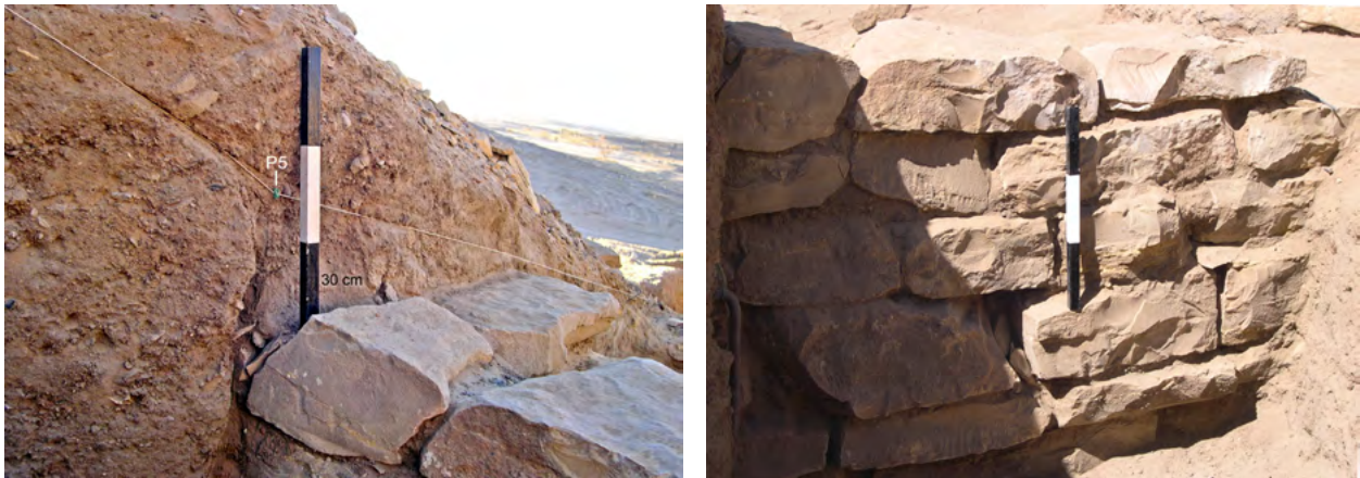
Figure 56. Sabaean Wall F4: details of masonry emphasizing the morphology and workmanship of the individual blocks. Scale 30 cm. (P. Morlupi 2005 © MAIRY, adapted and optimized by F.G. Fedele 2020)
