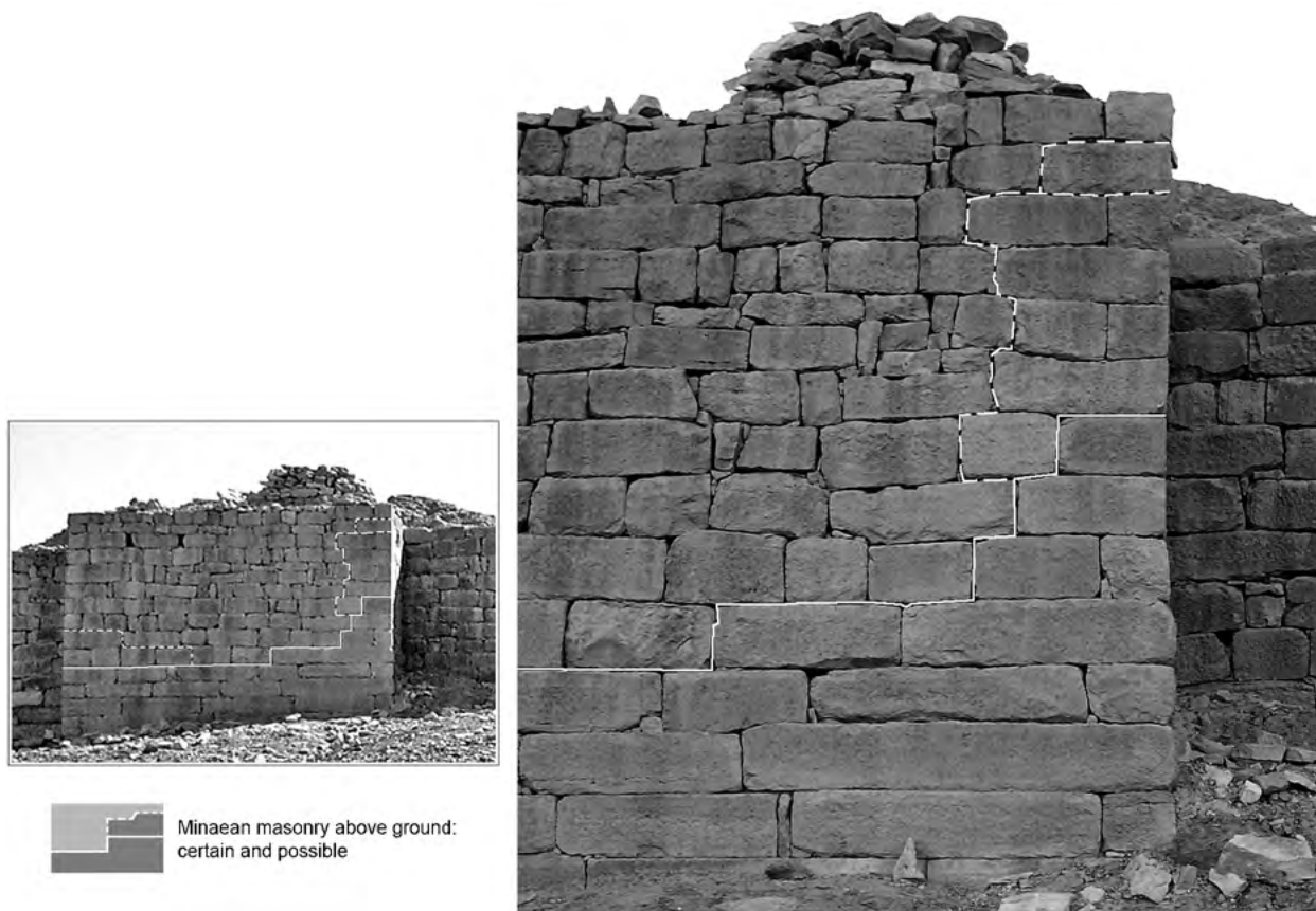
Figure 75. Minaean-Islamic wall: front views of bastion T7, suggesting the outline of the Minaean masonry above ground. (F.G. Fedele from photographs by P. Morlupi 2005 © MAIRY)
