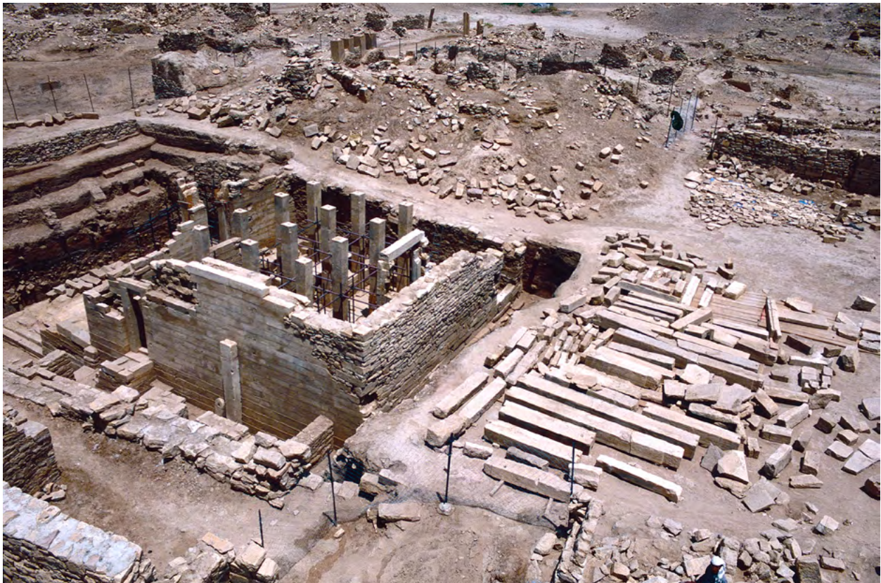
Figure 40. View of the temple of Nakrah from the crane arm: the temple's roof has been disassembled and the beams have been laid down on the southeast side of the building. (A. de Maigret 1992 © MAIRY)
