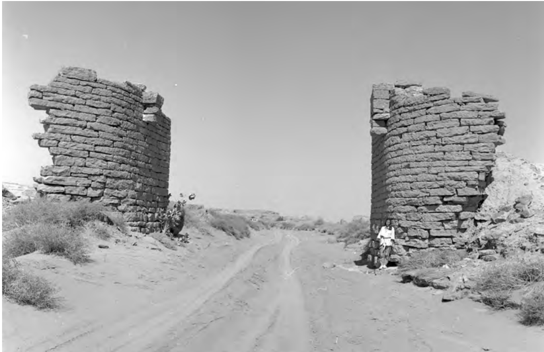
Figure 32. A monumental hydraulic structure in Wādī Shaqab, today reportedly destroyed. (A. Solazzi 1986 © MAIRY)
