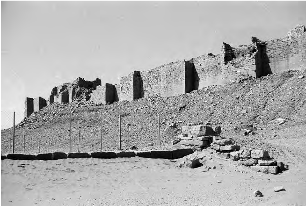
Figure 26. The weir to the east of Barāqish: the western wall. (A. Solazzi 1986 © MAIRY)
