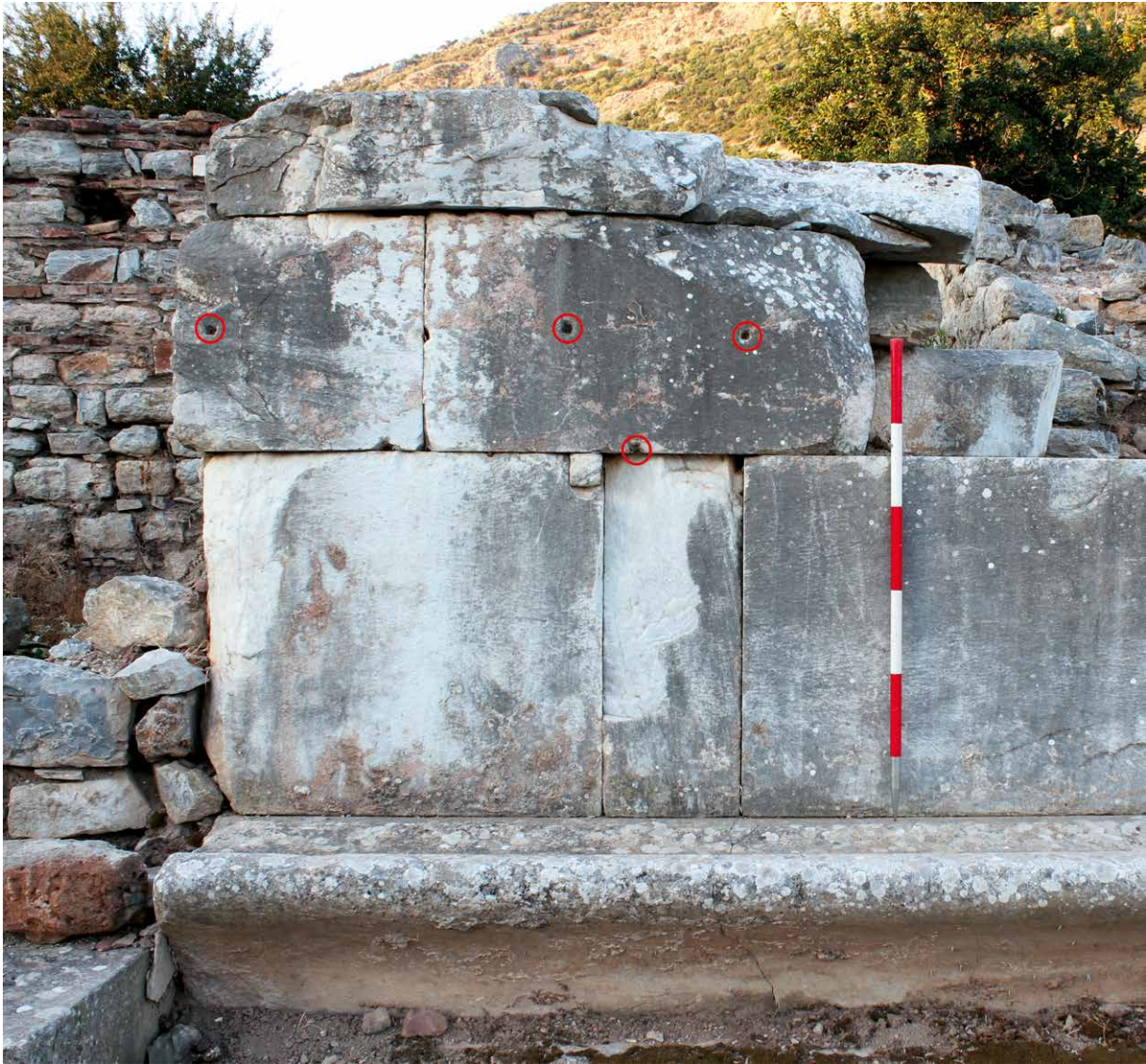
Figure 9. Ephesos, Upper Agora. South Stoa, section of back wall, with dowel holes (photo: Dirk Steuernagel, 2015).
