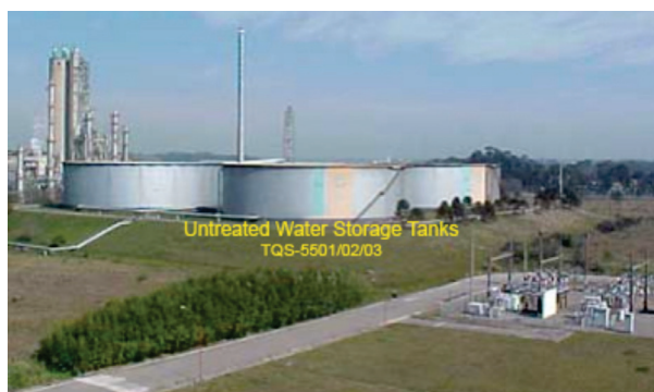
FIGURE 14 – UNTREATED WATER STORAGE TANKS OF REPAR REFINERY
