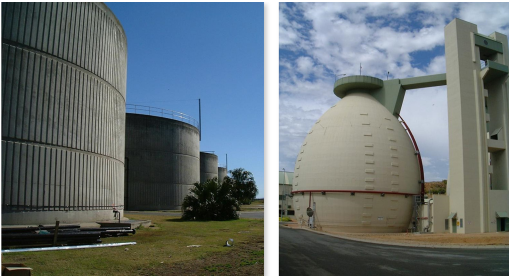
Figure 5.8 Examples of mixed liquor anaerobic digesters installed at municipal wastewater treatment plants in Australia.
