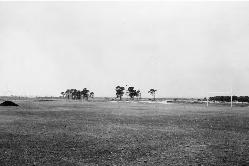
Figure 7.4: Goal posts erected after swamp ‘clearance’.
