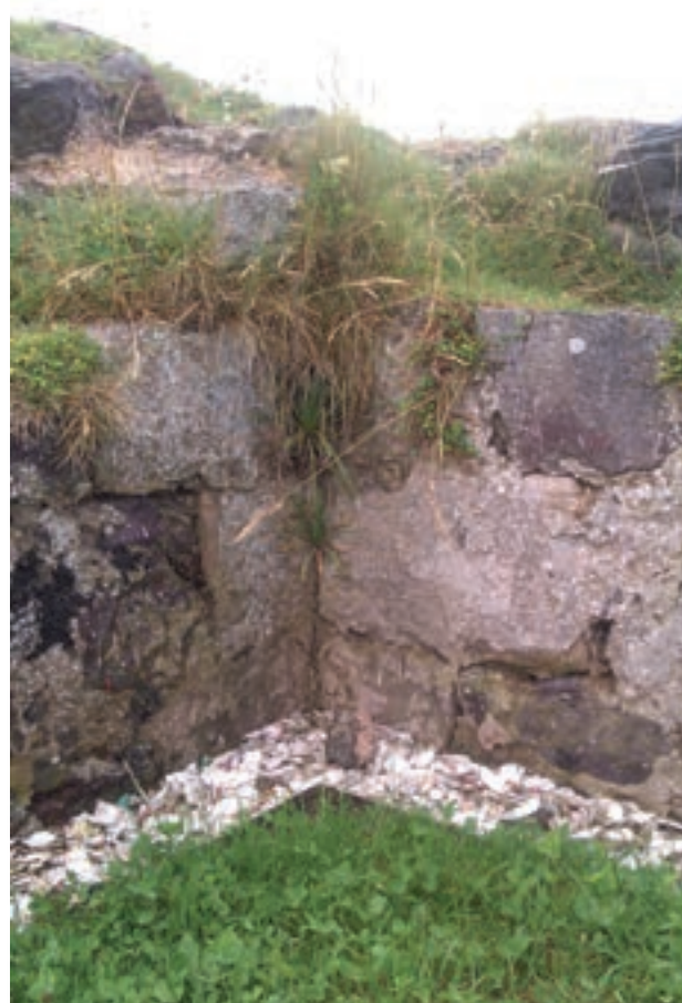
Fig. 4.25: North transept: dressed freestone blocks defining the internal re-entrant of its north and west walls – a diagnostically early feature, looking NW
