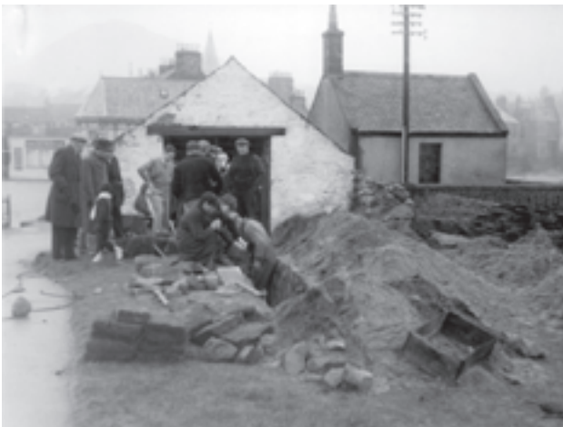
Fig. 4.17: View looking south, showing some of the building debris and monument fragments generated by the excavation (courtesy of Mrs Lorna Burton)
