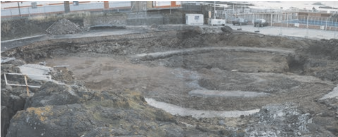
Fig. 1.5: General view of the Scottish Seabird Centre construction area, looking NW
