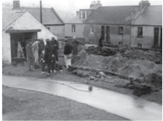
Fig. 4.16: The test trenching operation nearing completion, looking SW (courtesy of Mrs Lorna Burton)
