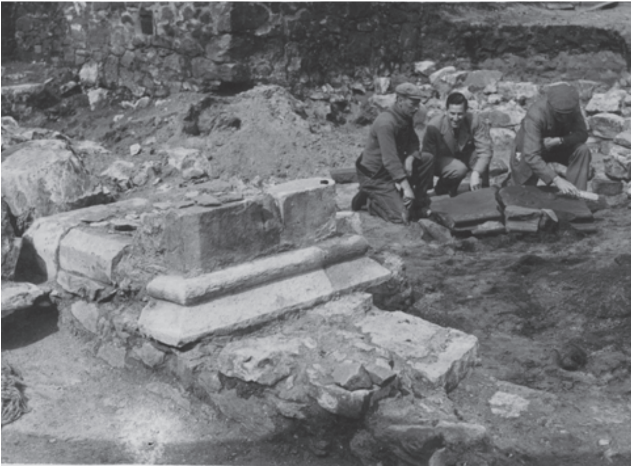
Fig. 4.21: The SW angle of the nave, left foreground, as newly revealed by the 1951 excavation, looking NW. The chamfered base course, which can be clearly seen forming the angle, has been cut through and overlain by the moulded pier base of the inserted nave arcade (Courtesy of East Lothian Council Archives & Local History Service).
