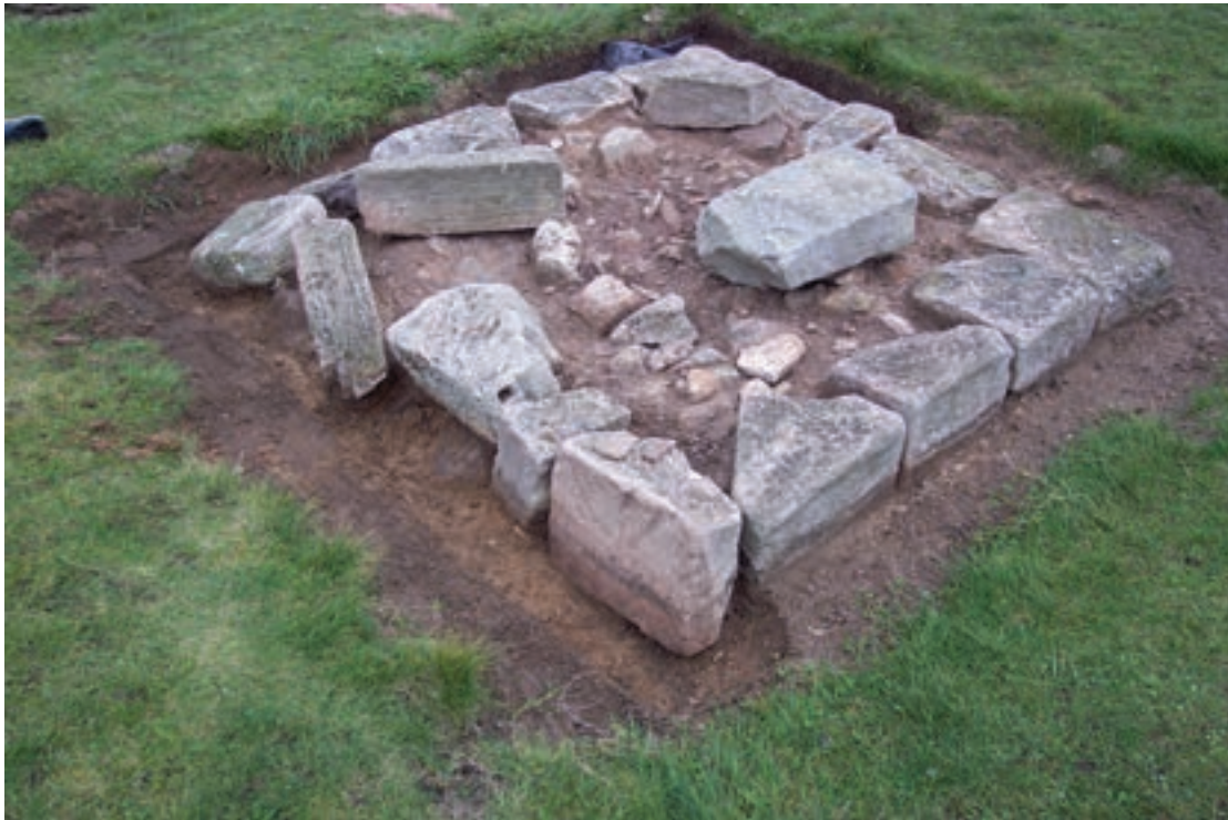
Fig. 4.26: Font base photographed from the SW, recorded during repair works in 2004
