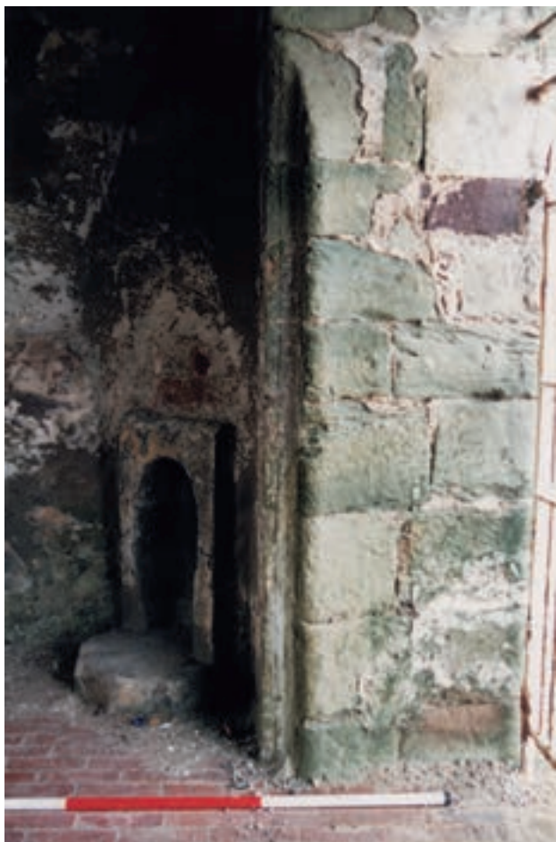
Fig. 4.27: The western jamb of the south entrance to the church preserved within the upstanding porch (note the fireplace and chimney breast above, inserted in the 19th century)
