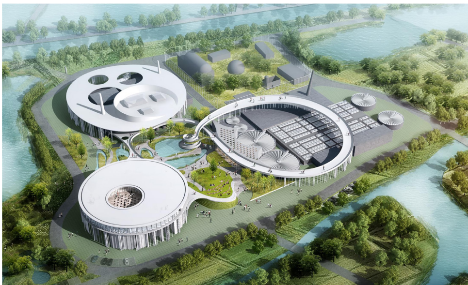
Figure 15.7 Yixing wastewater resource concept plant.
