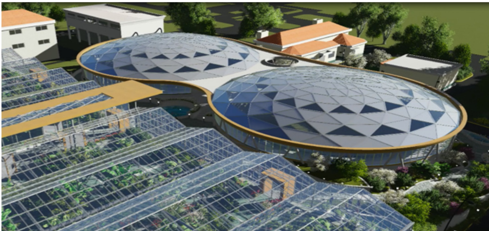
Figure 17.4 Wusong WWTF, image courtesy of Organica Water.
