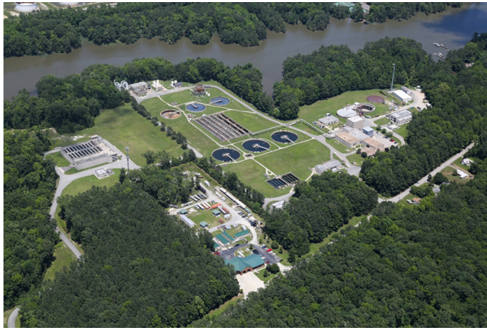
Figure 7.4 The Hampton Roads Sanitation District (HRSD) York River Treatment Plant (YRTP) in Seaford, VA.
