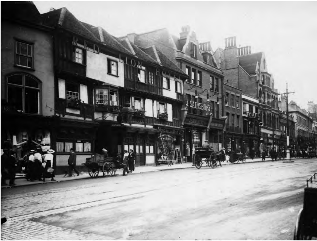
Fig 11.4 The Red Lion Hotel dates to 1515. It is probably the most significant surviving timber-framed building in Colchester (Colchester Museums).
