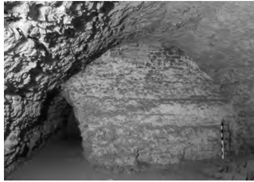
Fig 6.2 The 'vaults' or foundations of the Temple of Claudius as these appear today; the sand, which originally filled the void was dug out in the late 17th century (Colchester Museums).
