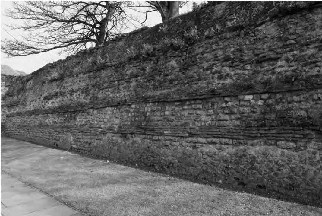
Fig 7.3 The Roman town wall to the south of the Balcerne Gate displays characteristic alternating courses of tile and septaria (Tony Nichols).
