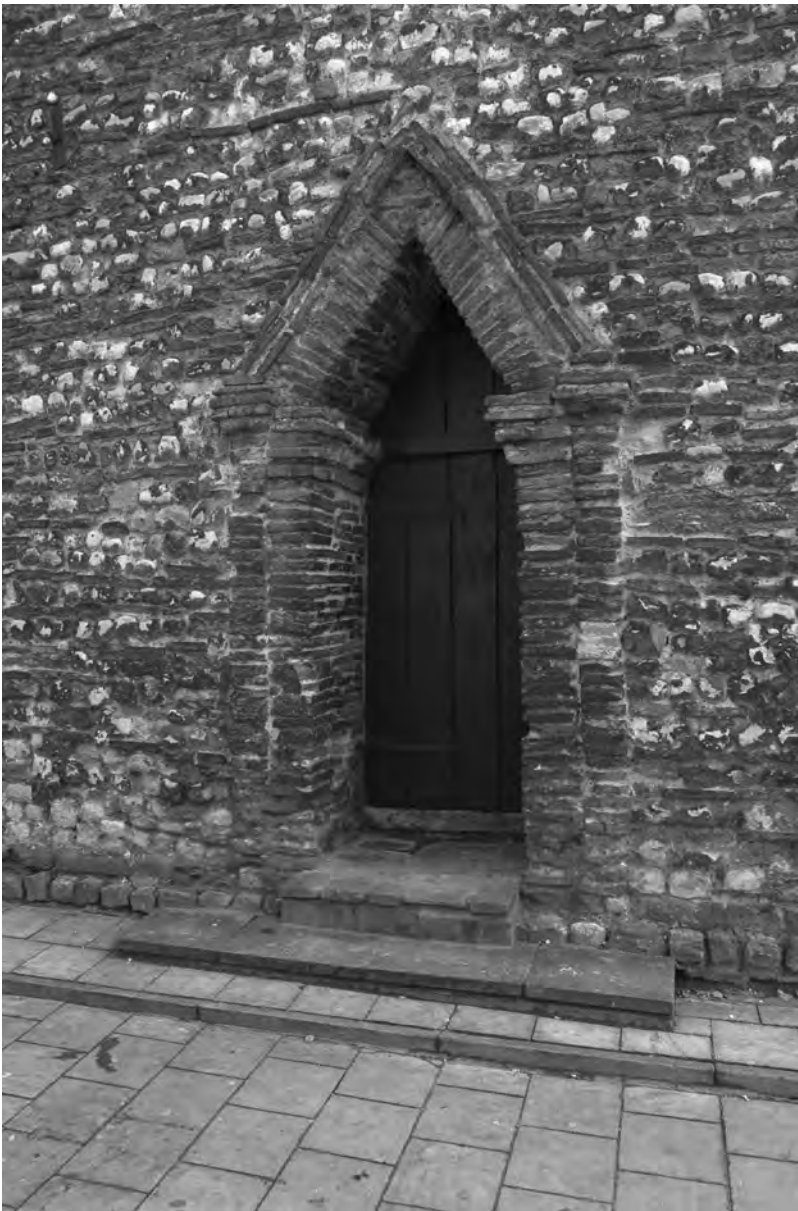
Fig 9.3 The triangular-headed west doorway of Holy Trinity church tower is of characteristic Anglo-Saxon design (Tony Nichols).
