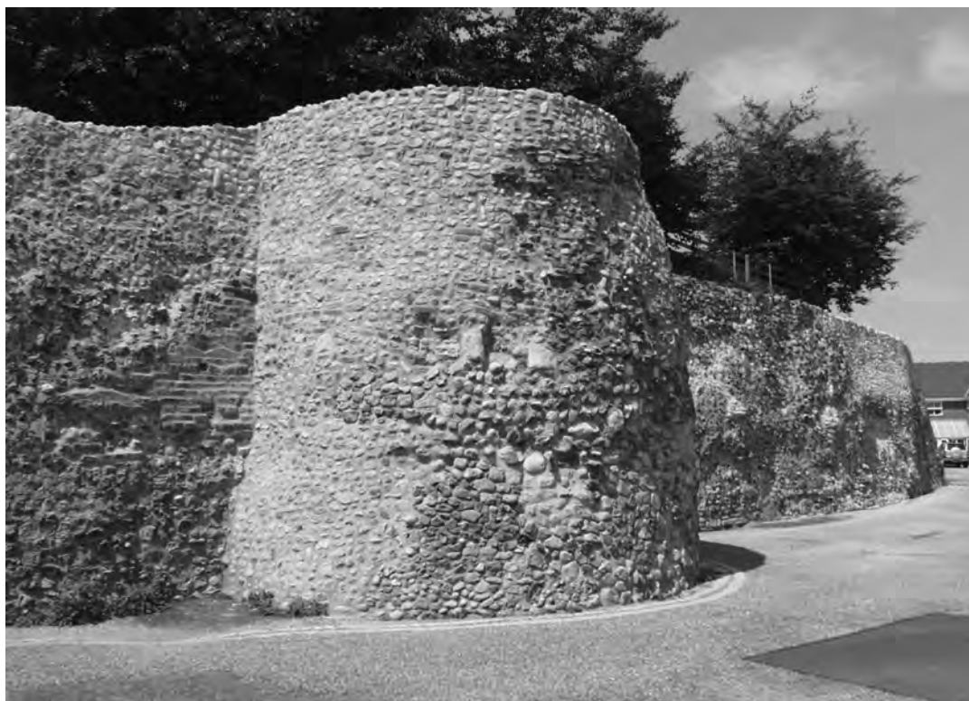
Fig 11.3 Bastion 2 in Priory Street is one of a series of external towers added to the town wall to strengthen its south-eastern corner (Philip J Wise).
