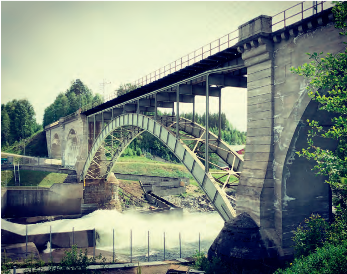
Figure 1: Sikfors railway bridge in Sweden, built in 1912, presents an example of steel structures that need anticorrosive paint treatments. Photograph by Sven-Olof Ahlberg.
