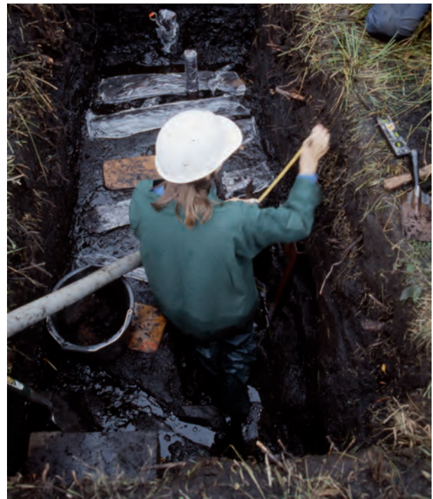
Figure 22. Excavations of the Sweet Track for condition assessment.
