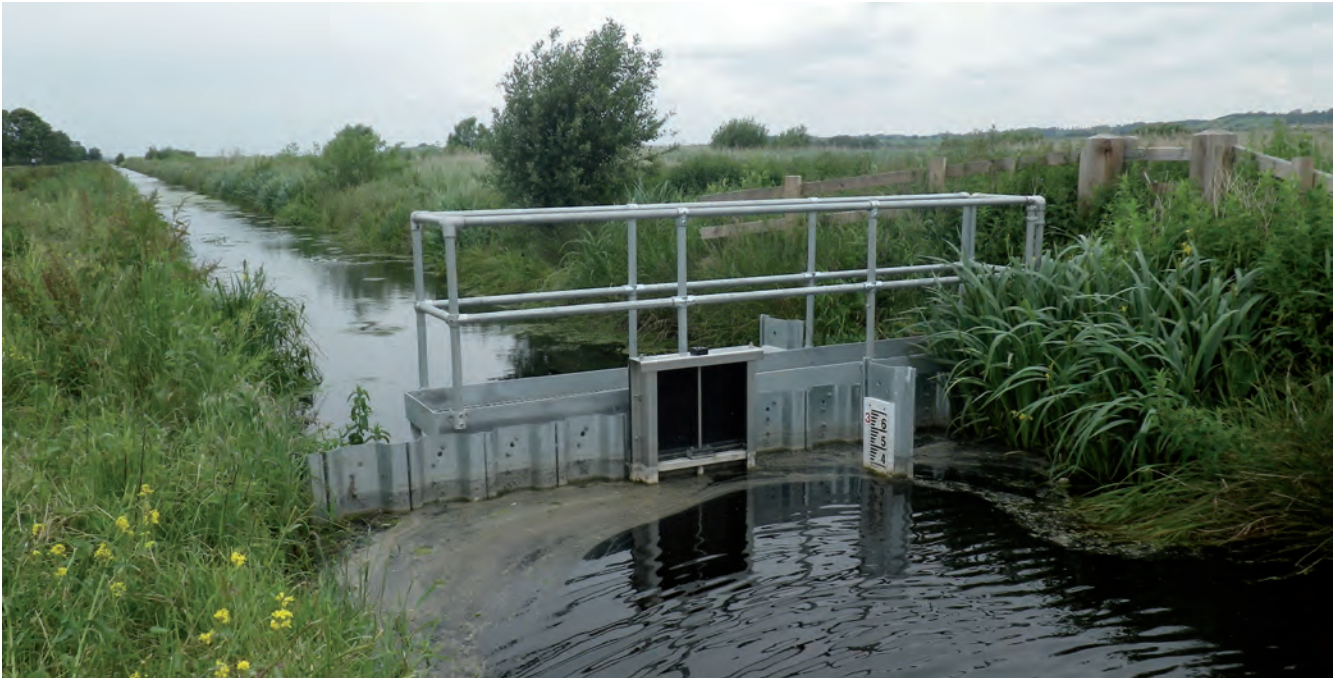
Figure 217. New weir structure.
