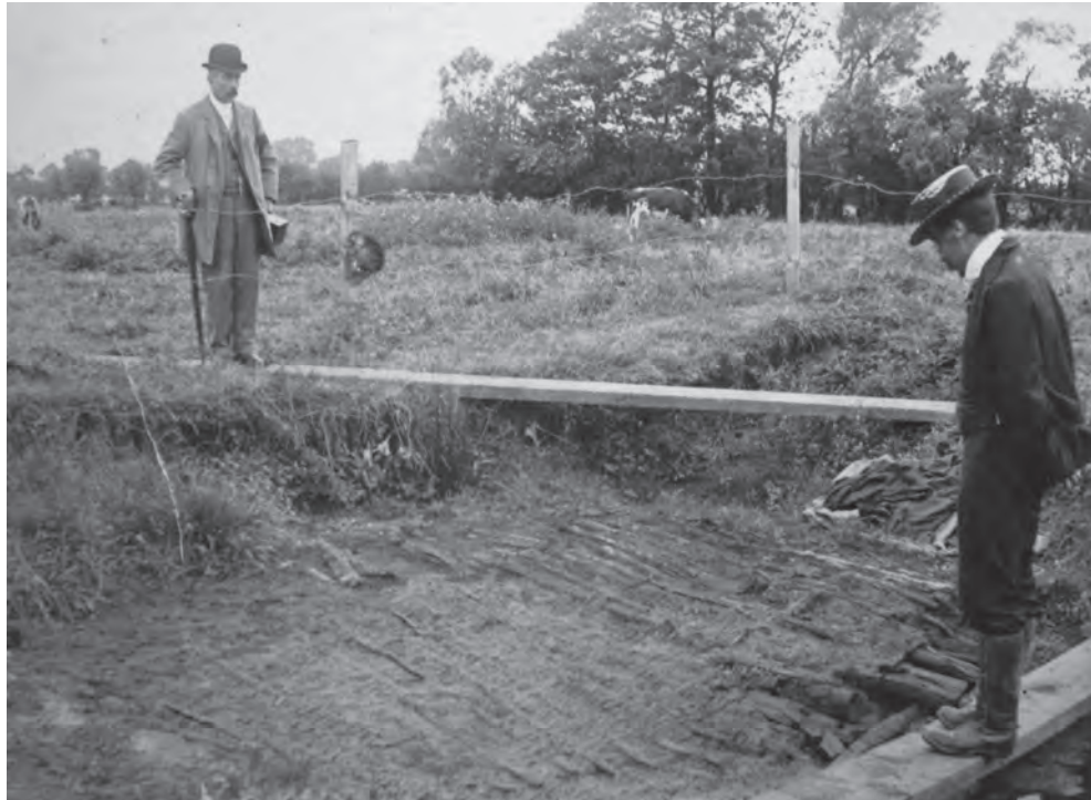
Figure 153. Wattle panel in the foundations of the settlement revealed in the Bulleid and Gray excavations (Bulleid on right).
