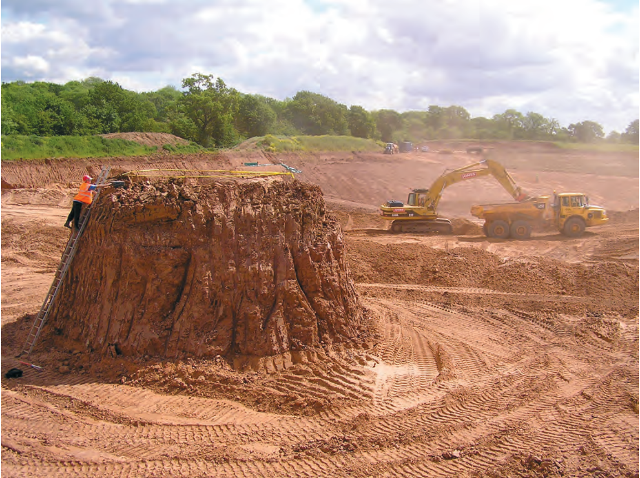
Fig. 5.14 Archaeologists fence off an area of Late Iron Age settlement during topsoil stripping at Bubbenhall Quarry; the quarry operator removes surrounding overburden and provides ladder!
