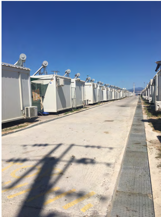
12.4 Containers/prefabricated housing units, Skaramangas camp (the largest camp in mainland Greece, located on a dock of the Hellenic navy, in a shipyard area), Attica, May 2020. © Nada Ghandour-Demiri.
