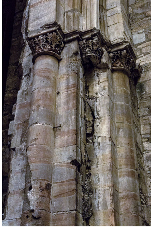
Fig. 2: Church of St Reinold, Dortmund, clustered pillars in front of western nave wall; traces of wartime destruction left as a reminder; photo: Allegra Höltge, Department of Fine Arts, TU Dortmund University
