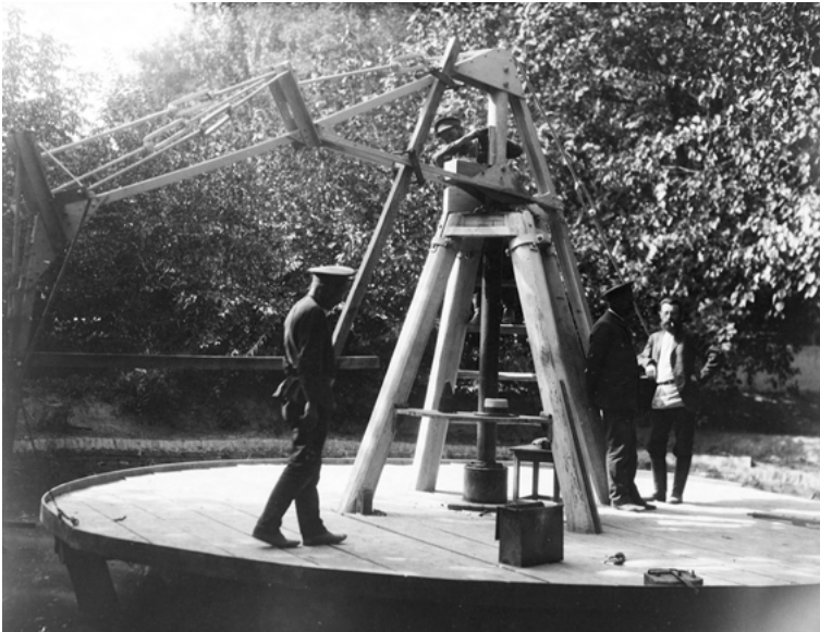
Figure 7.12: “A station for checking water velocimeters. Tashkent”. September 7, 1912. GBU “TsGAM”. N. M. Shchapov’s archival collection. 2-2380.
