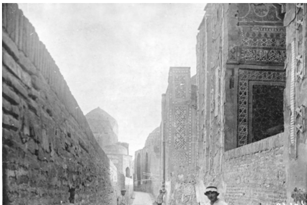
Figure 11.3: “Corridor of the central group of mausoleums, Shah-i Zinda, Samarkand, taken during the Turkestan architectural expedition of 1921”. Archive of the Institute for the History of Material Culture, Russian Academy of Sciences.
