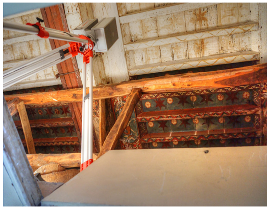
Fig. 05. Left: the scanner viewed from the trapdoor and the part of the ceiling covered by a white coat. Right: the station points for the laser scanning survey of the ceiling (Authors' image).
